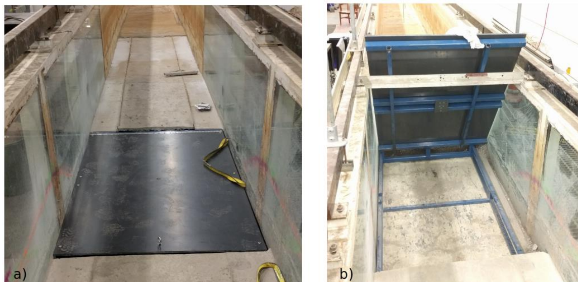
Figure 4-5: Pressure board. (a) Final installation inside the existing bathymetry; (b) Example of the hinge mechanism and bottom access.
