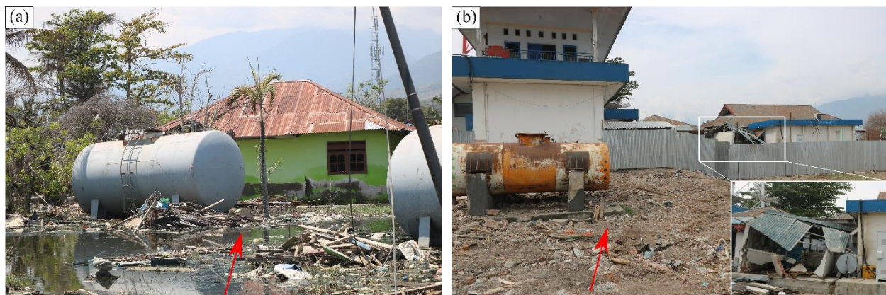
Fig. B - 4. APST transport and impact on structures from (a) Palu Gas Station and (b) TVRI Palu. The approximate primary flow direction is indicated with a red arrow.
