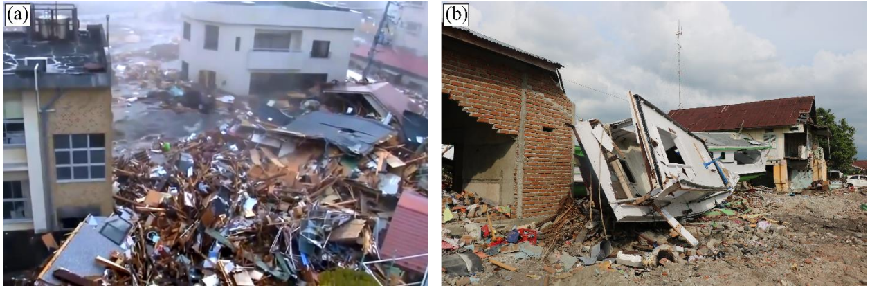
Fig. 2-5. Field evidence of debris damming loads in (a) the 2011 Tohoku Tsunami (YouTube, 2011) and (b) the 2018 Palu Indonesian Tsunami.
