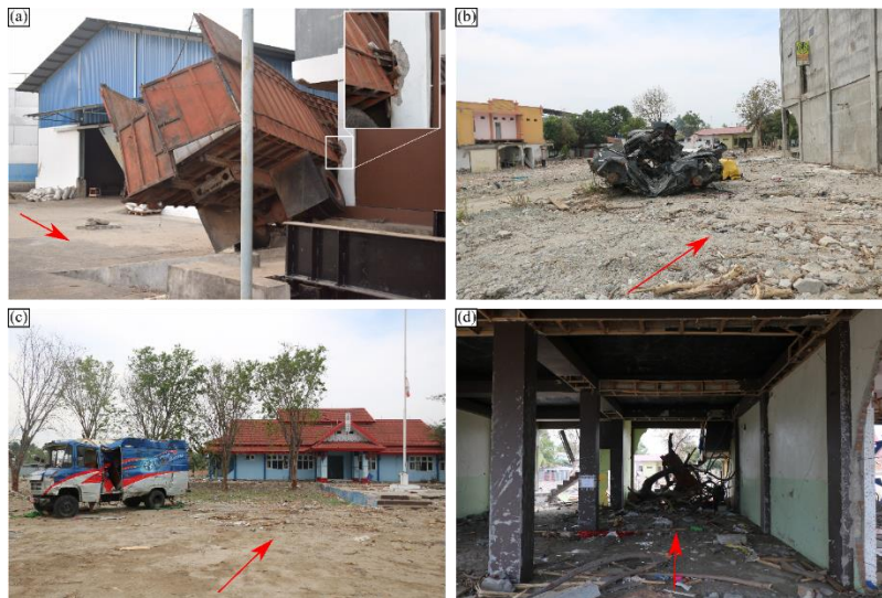
Fig. B - 7. Vehicle impacts at (a) Mamboro Fuel Station, (b) TotalX, and (c) TVRI Palu. (d) Debris damage to internal structural columns observed at TotalX. The approximate primary flow direction is indicated with a red arrow.
