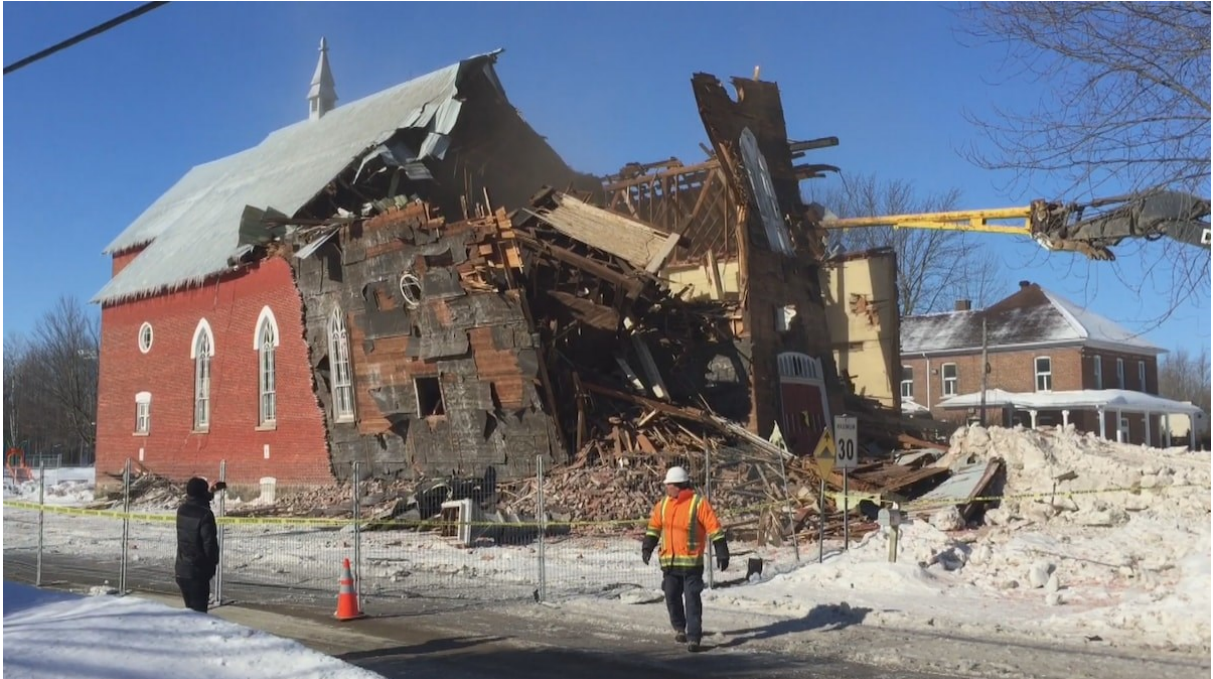
Figure 8 The Demolition of Saint-Edmond-de-Grantham
