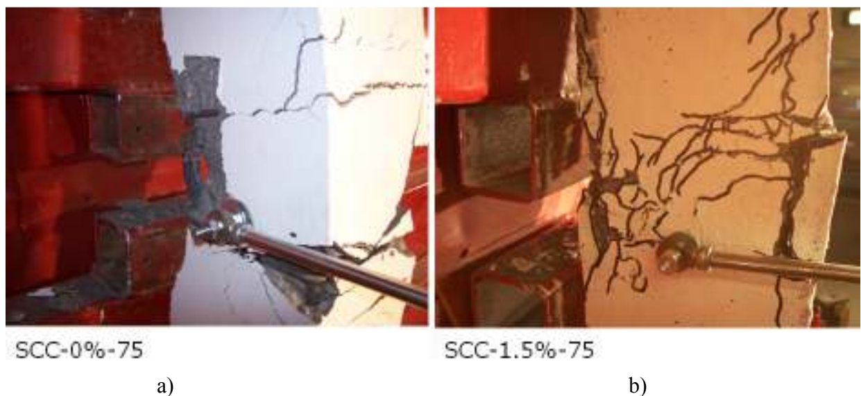
Figure 5.3 Comparison of the mid-span after Blast 3 of a) SCC-0%-75 and b) SCC-1.5%-75
