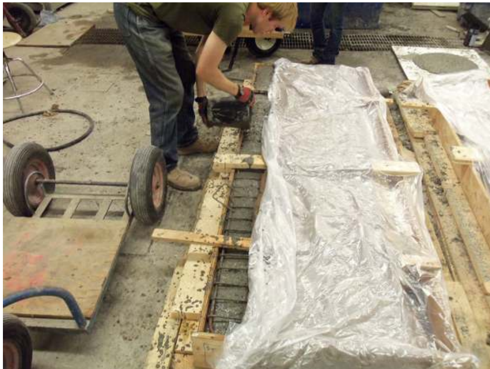
Figure 3.9 Placing concrete and curing the columns
