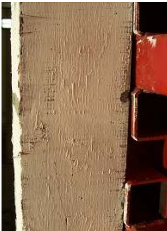
(a) Mid-Span Result of Blast 2
