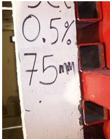
(b) Chipping of concrete
