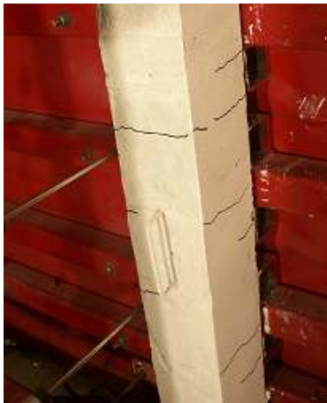
(a) Mid-Span Result of Blast 1
