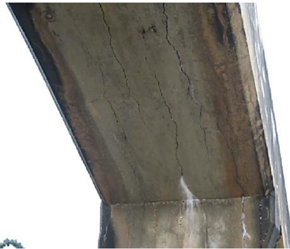
Figure 2.2: ASR-related signs in bridge elements [11,21].
