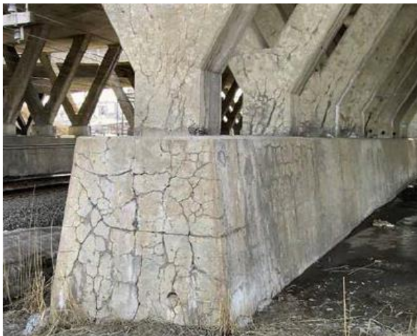
Figure 2.2: ASR-related signs in bridge elements [11,21].
