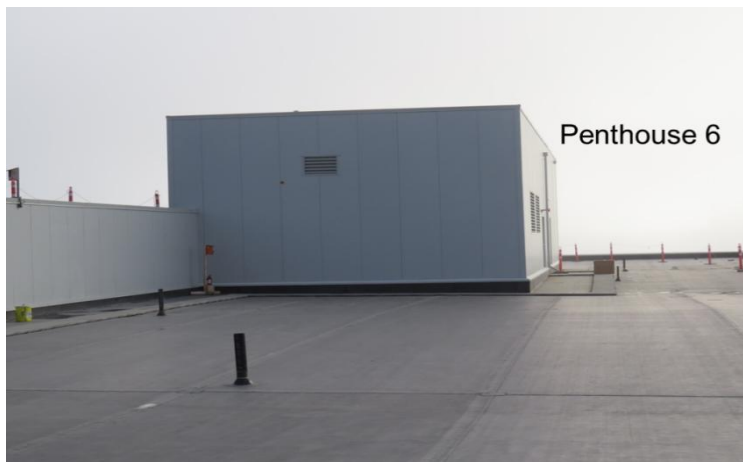
Figure 3.6: Close up of Penthouse 6 (Courtesy of NRCC)
