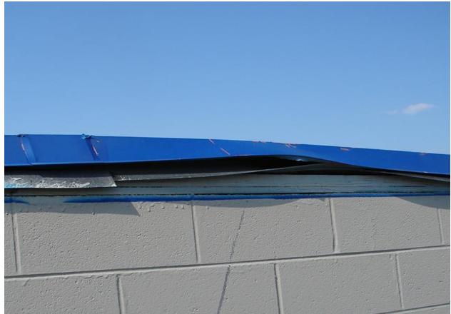
Figure 1.3: Typical roof edge failures during high wind conditions: (a) complete failure, (b) partial failure, (c) cleat failure and (d) coping failure. (Courtesy of NRCC)
