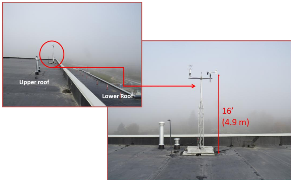
Figure 3.4: Wind tower installation at the upper roof level (Courtesy of NRCC)
