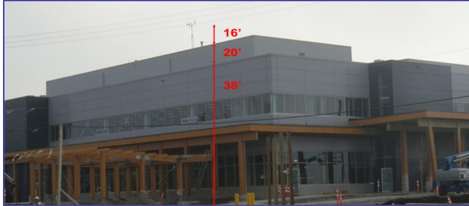
Figure 3.3: Elevations of the lower and upper roofs, and of the wind tower (Courtesy of NRCC)
