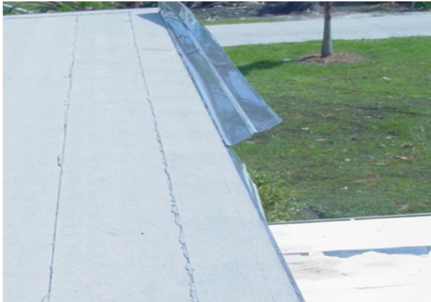
Figure 1.3: Typical roof edge failures during high wind conditions: (a) complete failure, (b) partial failure, (c) cleat failure and (d) coping failure. (Courtesy of NRCC)
