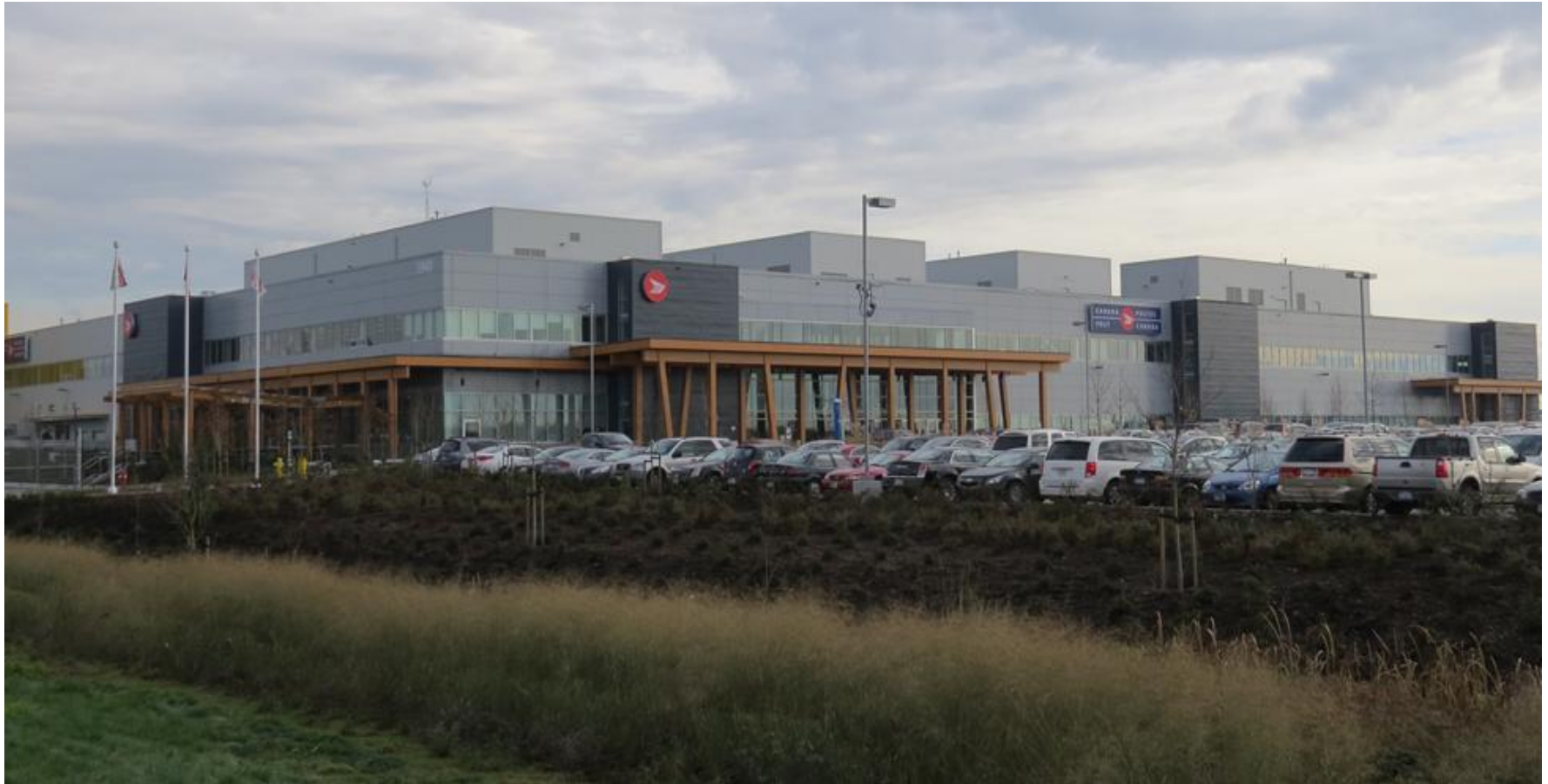
Figure 3.1: Canada post building in Vancouver, Canada (Courtesy of NRCC)
