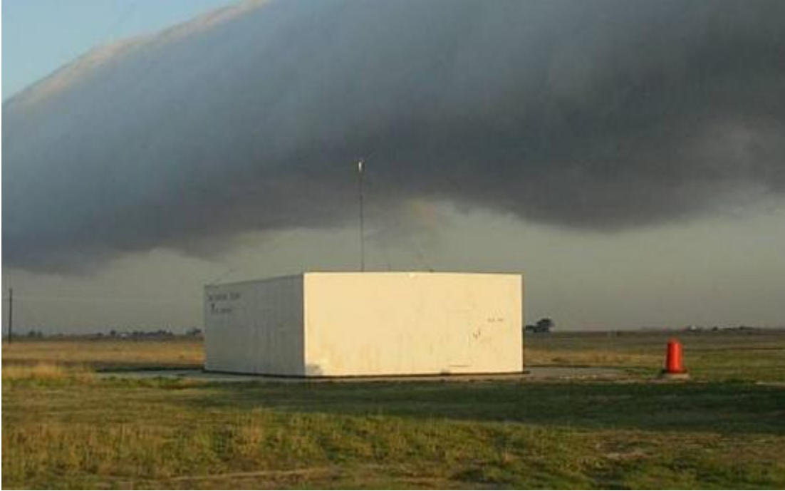
Figure 2.8: Wind Engineering Research Field Laboratory (WERFL) test building ( https://www.depts.ttu.edu/nwi/facilities/WERFL.php .)
