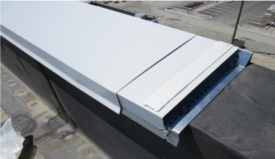
Figure 3.12: Anchor Clip splice plates with pre-applied adhesive tapes (Courtesy of NRCC)
