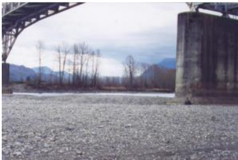
Fig. 1-1. Bridge pier scour at the Agassiz Bridge in the Fraser River, B.C. from Valela et al. (2018).
