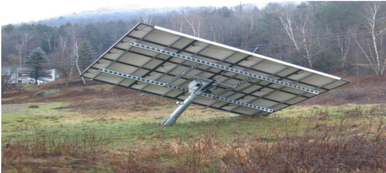
Figure 1.1: Damaged of ground mounted PV tracker in Northern VT, U.S.A. [9]
