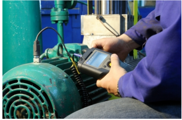
(b) Measuring vibration with a vibration meter 2
