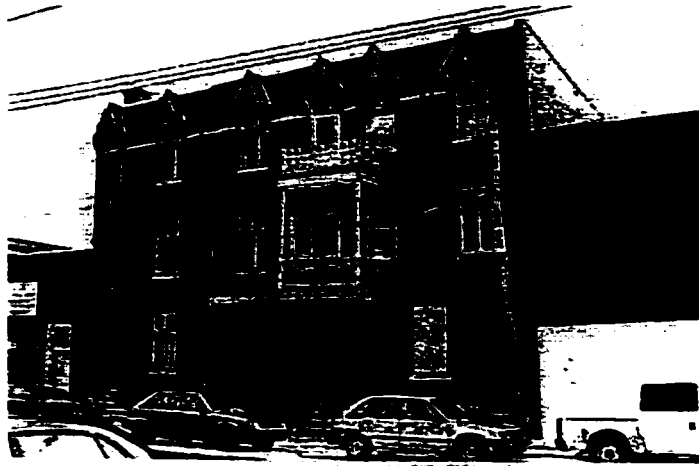
Figure 5.1 Three-story older residential building in Montreal, Canada from which wall specimens were retrieved.
