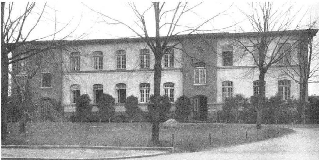
Figure 1: Photography of one of the original houses constructed (around 1900). 6
