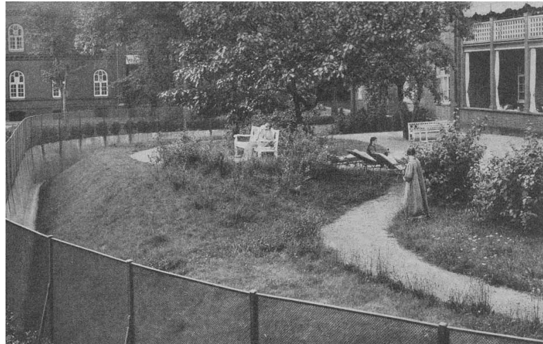
Figure 24: View on the secure House 8, c. 1928. Note the construction of the fences flush to the ground. 2
