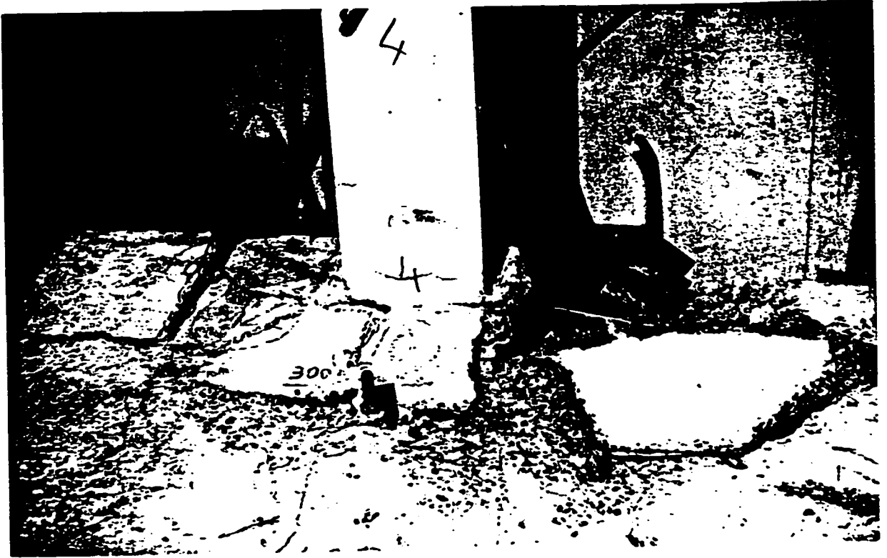
Fig. 4.25 The severe damage of connection no. 4 due to punching shear failure in Test no. 4
