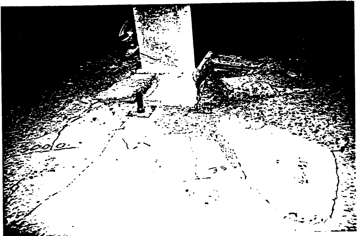
Fig. 4.4 Punching shear failure zone at column no. 2 in Test no. 1
