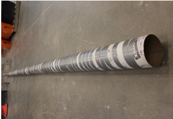
Stage 3. Connecting Sonotubes segments together
