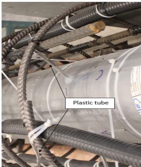
Extension wires attached to the sonotube
