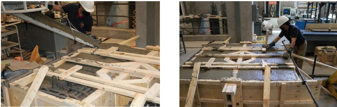
Figure 3.21. Pouring the concrete in the formwork
