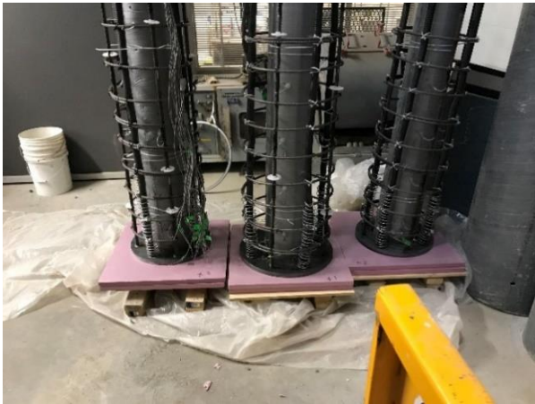
Styrofoam sheets underneath the towers' base
