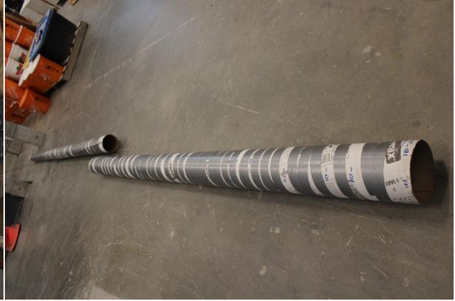
Stage 2. Rolling Sonotubes to the proper tapered shape
