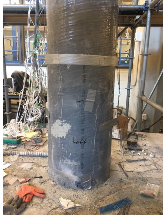
(b) Sides of the towers' surface
