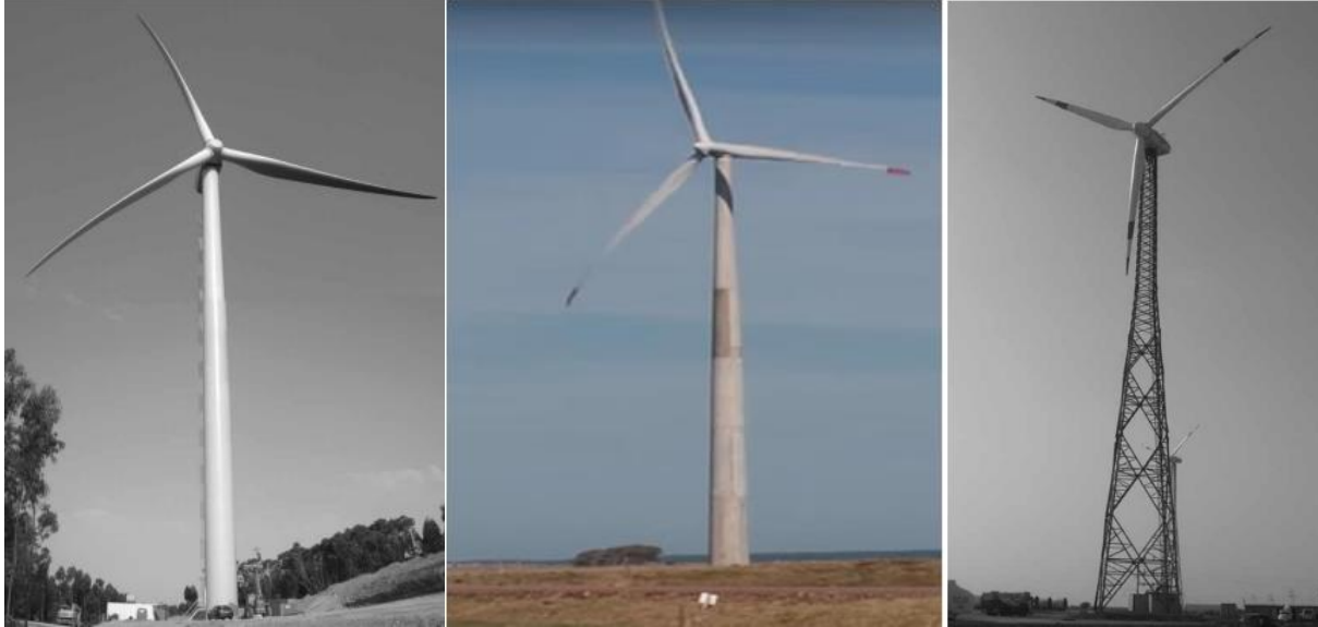
Figure 2.1. (a) Steel tubular tower (Veljkovic et al., 2011), (b) Concrete tower (ACCIONA, n.d.), (c) Steel lattice tower (Veljkovic et al., 2011)
