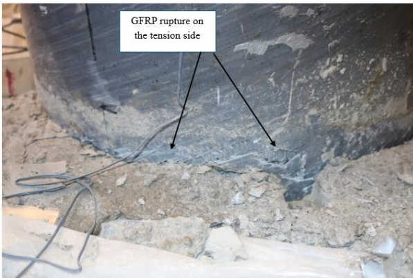
(c) FRP tensile rupture above the foundation block
