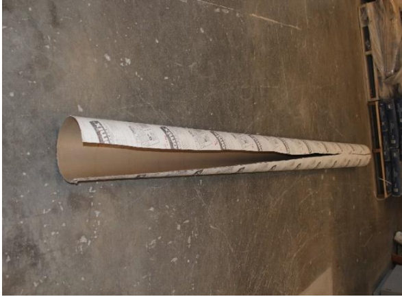
Stage 1. Cutting Sonotubes to the required diameters
