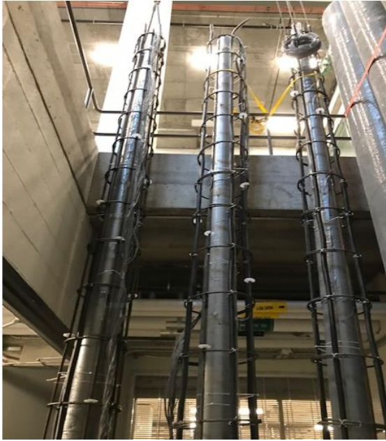
Steel cages before placing the GFRP tubes on them
