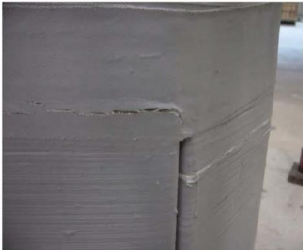
Shear rupture of specimen P3-1
