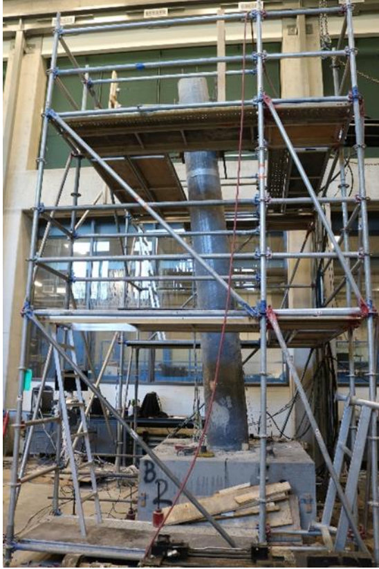
(a) Tower at ultimate displacement
