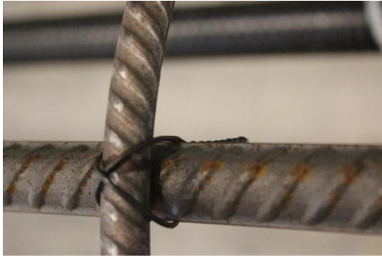
Steel bars secured to ties at marked locations
