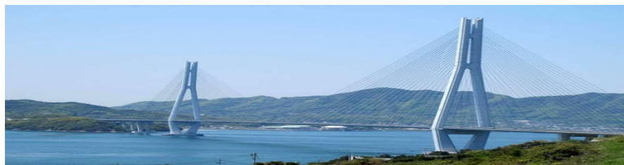
Figure 1-2: Tatara Bridge, main span of 890 m [3]
