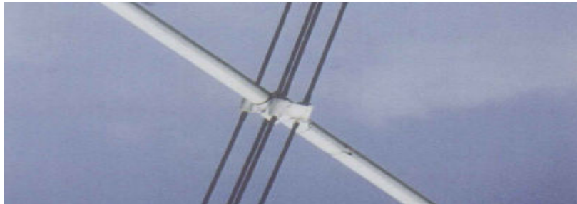
Figure 2-5: Detail of cable clip on Normandy Bridge [2]
