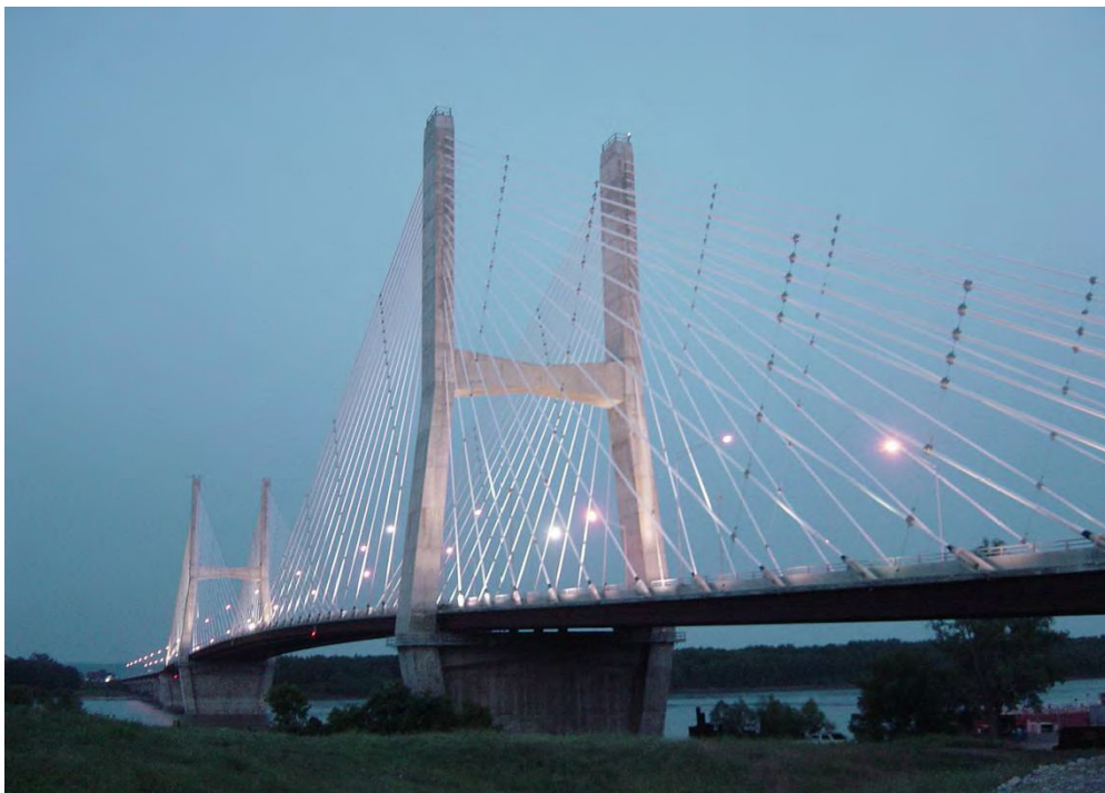
Figure 3-35: Joint points of Crossties of Bill Emerson Memorial Bridge [10]
