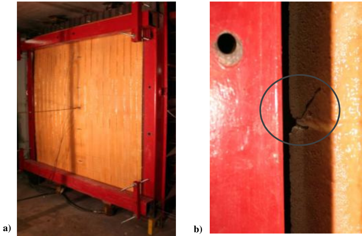
Figure 3.61: Retrofitted Load-Bearing Wall URM-4: a) After Shot 6; b) Tension Cracks Developed Near the Middle Mortar Joint after Shot 6
