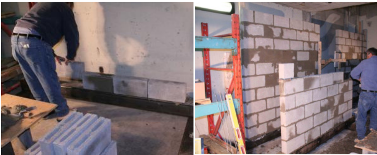
Figure 2.7: Standard 100 \times 200 \times 400 Concrete Masonry Unit Block (Glanville et al., 1996)
