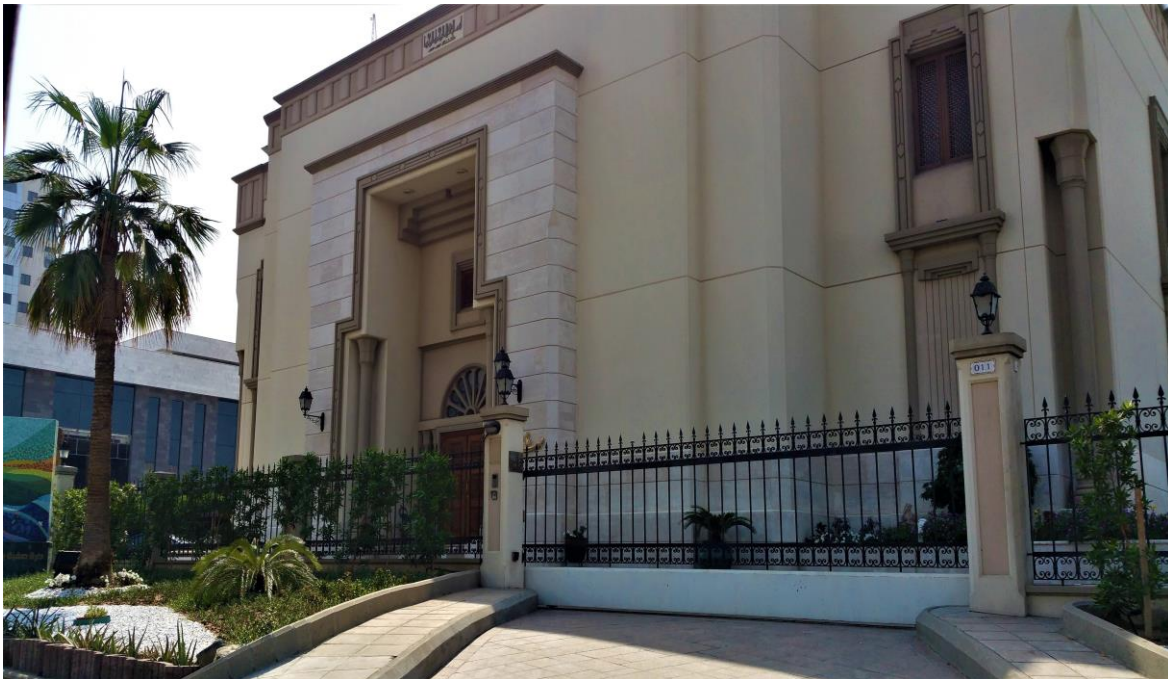
Figure 5:12: The entrance of “Darat Safeya Binzagr”
