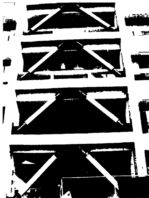
Figure 2.20: Retrofit scheme during construction, BRBF (Skokan et al. 2010)
