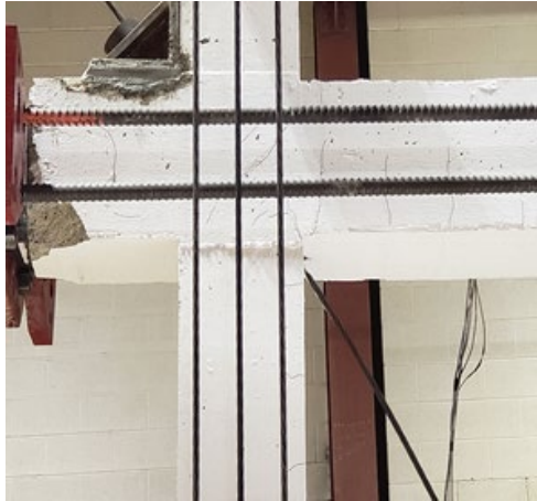
(a) West beam-column joint
