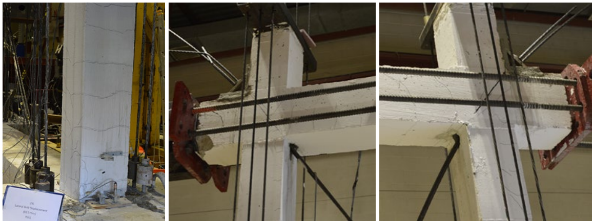
Figure III-4 crack pattern at the end of 2% drift cycles
