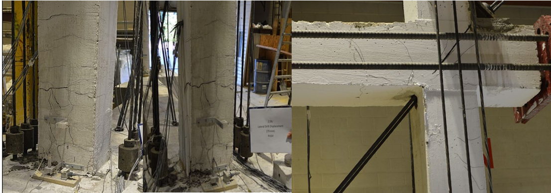
Figure III-5 Beginning of cover concrete crushing and crack pattern at 2.5% drift during Test 2
