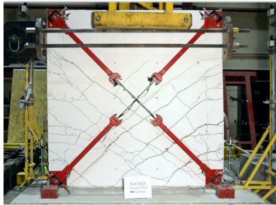
Figure 2-52 Non-ductile squat wall retrofitted by HSS and SMA braces (Cortés-Puentes and Palermo 2018)
