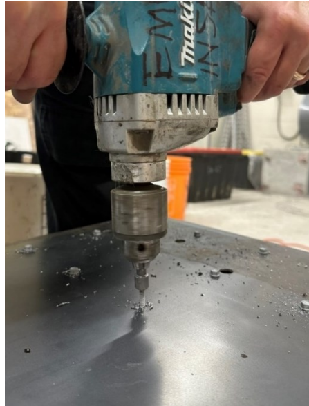
Figure 42: Self-drilling screw installation
