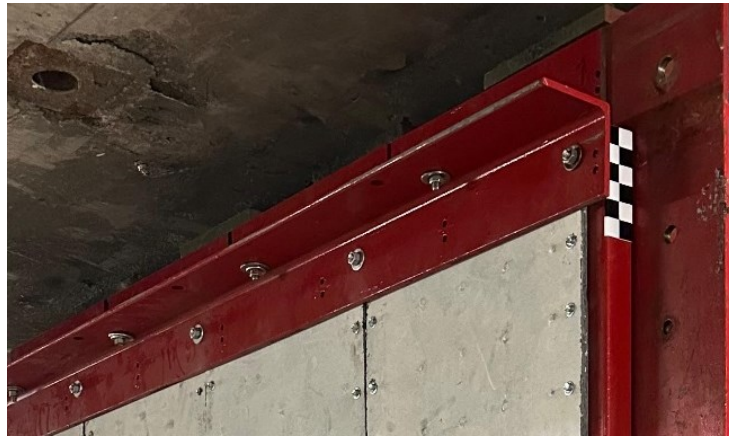
Figure 53: Support angles, HSS, and panel connection
