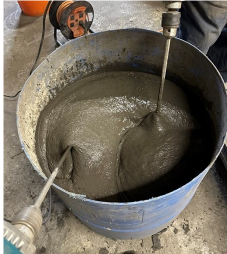
Figure 45: Two hand mixers are being used simultaneously for mixing in a plastic drum
