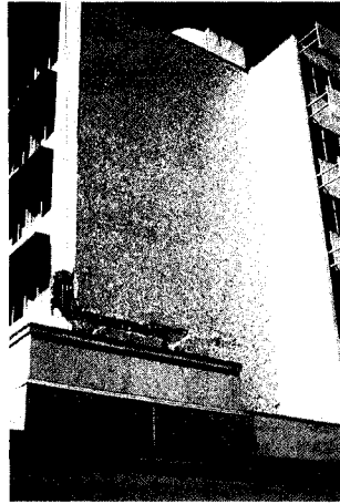
a) Holy Cross Building, Los Angeles, California, 1971 San Fernando Earthquake. Failure of this wall occurred at the fourth floor level during the earthquake due to poor workmanship.
