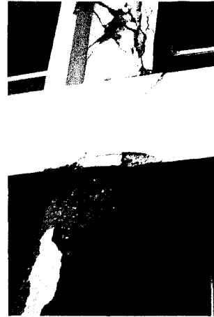
b) Illustrating clearly how the concrete in this critical region has been disrupted (broken off) as a consequence of the premature (early) ending of the spiral reinforcement.
