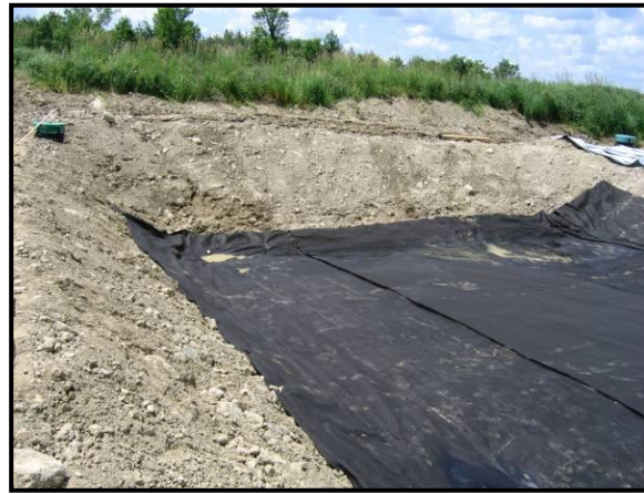
Geotextile laid out (2)
