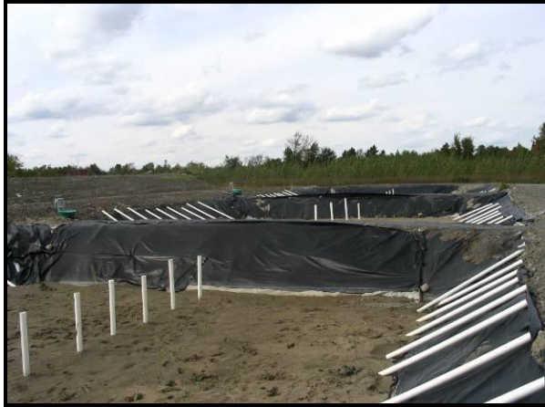
Geotextile to protect liner from UV rays (9)
