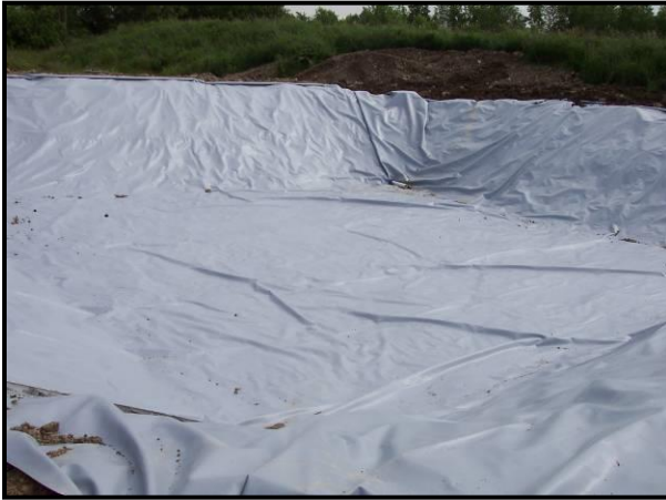
Liner laid out (5)
