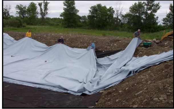
Unfolding the liner (4)
