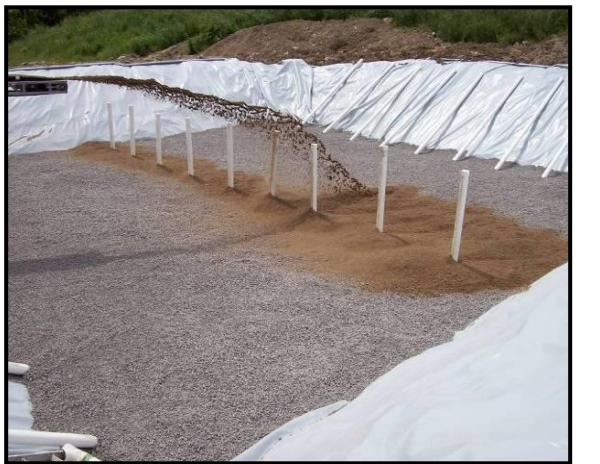
Placing Sand in Filter (8)
