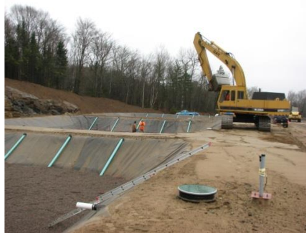
Figure 7-1. Plan View and Photo of Algonquin Park Septage Reed Bed System (Credit: Ontario Parks)
