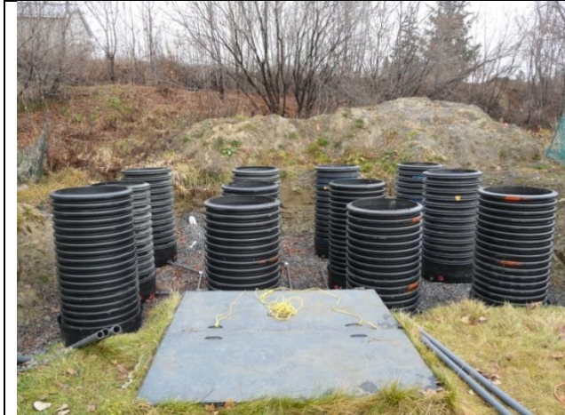
Pilot Filters before Backfilling
