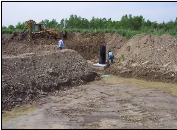
Installed pump chamber with excavated bed (1)
