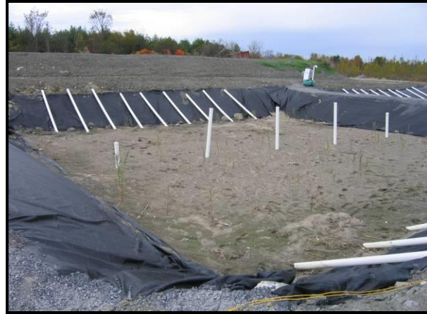
Completed filter with planted reeds (10)
