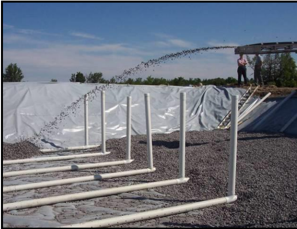
Placing gravel in base of filter (7)
