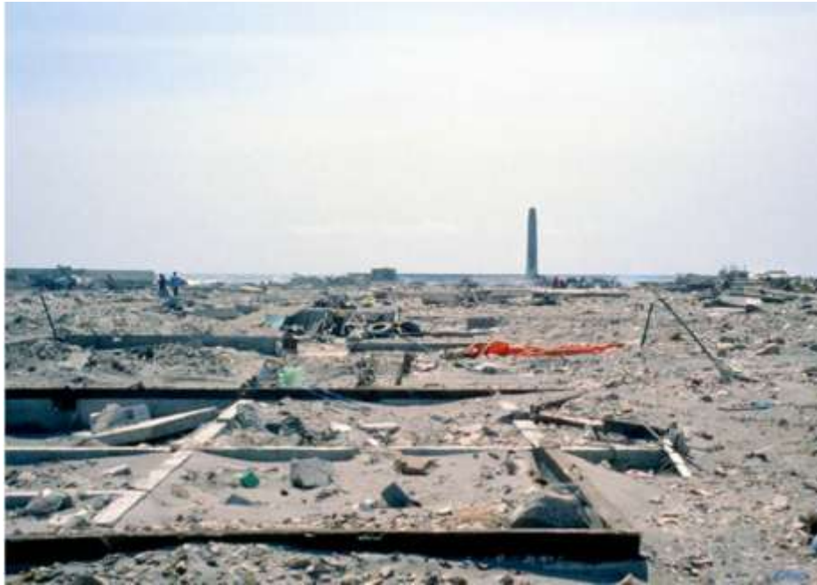
Figure 2:Damage caused by 1993 Okushiri Tsunami, Japan (FEMAp646a) Damage caused by 1993 Okushiri Tsunami, Japan (FEMAp646a)
