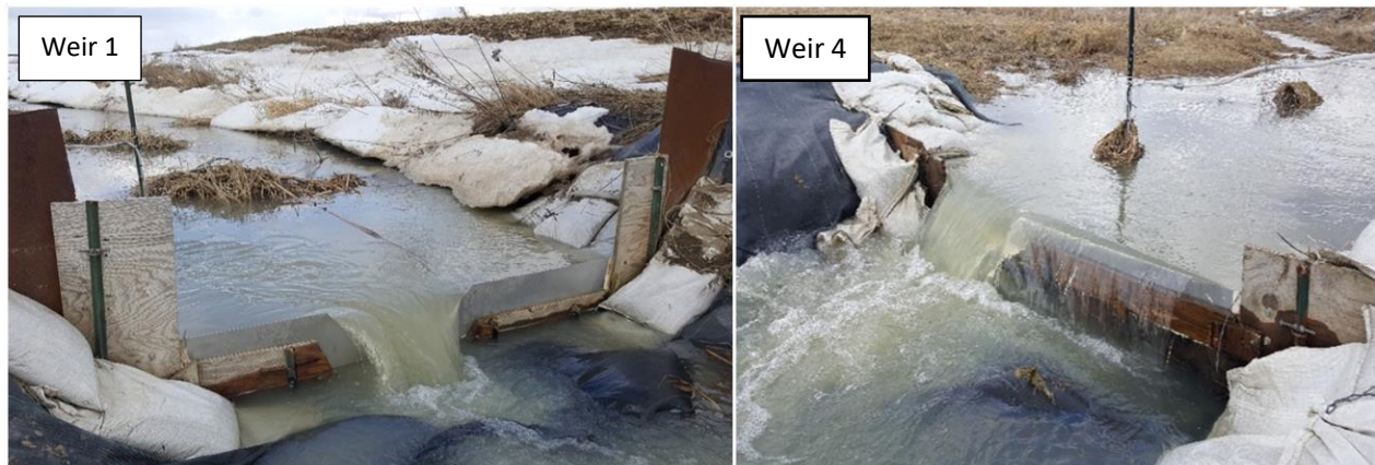
Figure 3.3: Left: Pond Inlet (Weir 1) and Right: Pond Outlet (Weir 4). These photographs were used with permission from Olatian Edu (2017 Water Budget Balance for Wetland in Bercier Farm).
