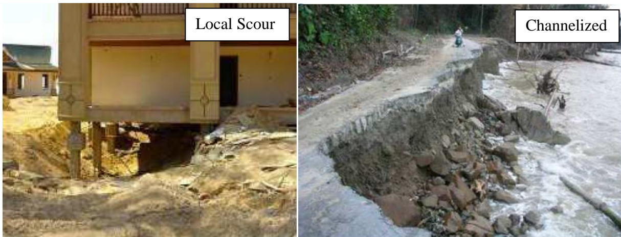
Figure 2.5: Types of scour mechanisms (Tonkin et al., 2013)
