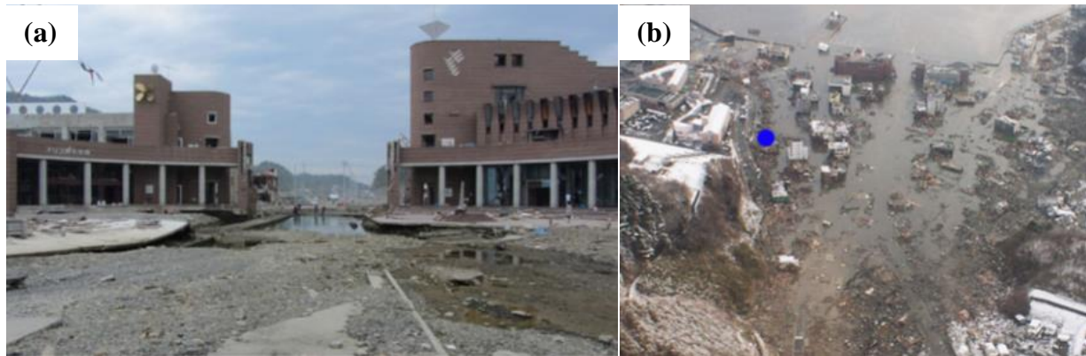
Figure 2.10: Channelized between two tsunami resistant critical infrastructures (a) View from shore side (b) Aerial view of the affected area (Yeh et al., 2013)
