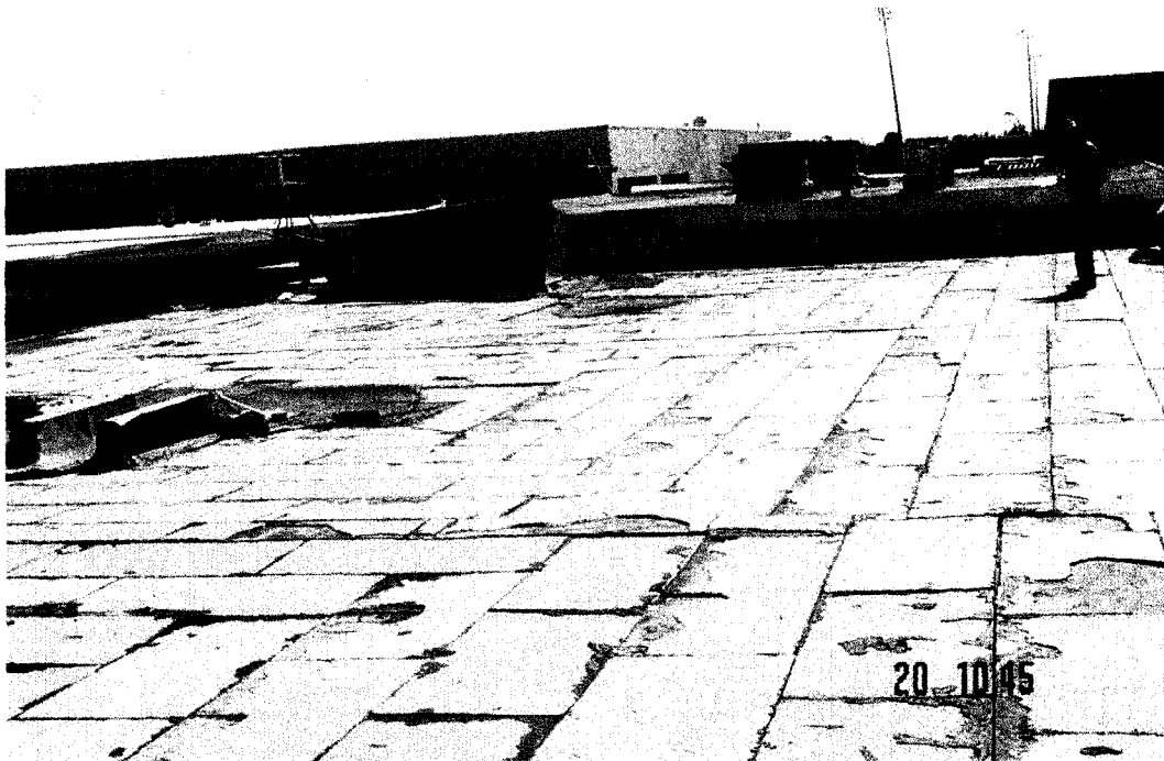
Figure 1.9: Wind Uplift Failure of Roofing System during Hurricane Charley (Baskaran et al, 2006)
