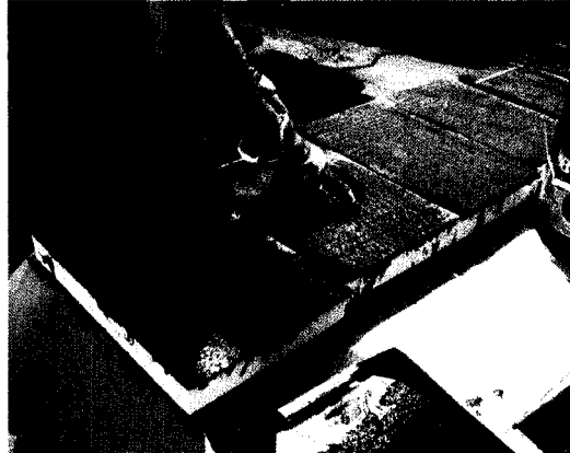
Figure 3.2h: Adhering base sheet
