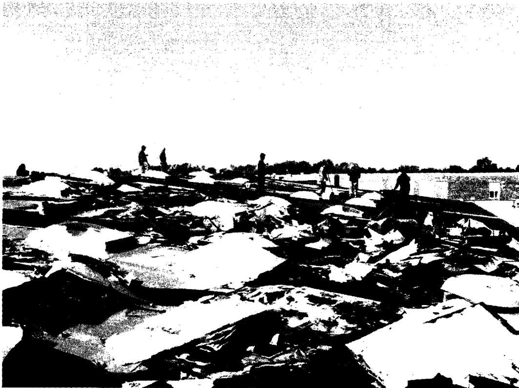
Figure 1.8: Wind Uplift Failure of Roofing System during Hurricane Charley (Baskaran et al, 2006)
