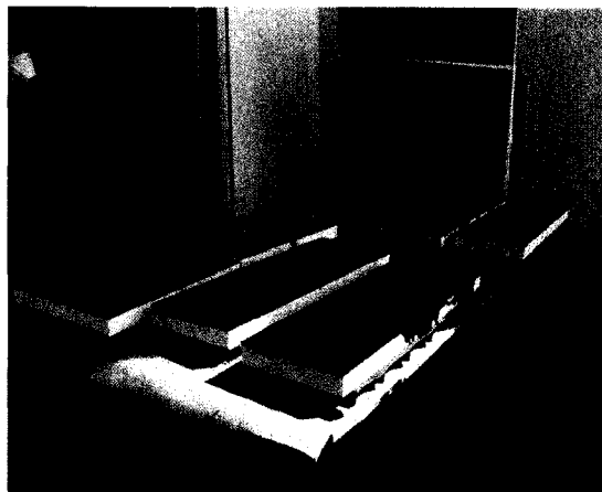
Figure 3.2f: Adhering coverboard
