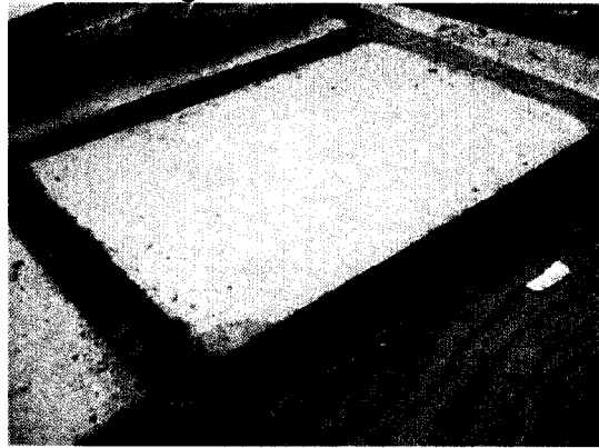
Figure 3.4d: Concrete slabs, final product
