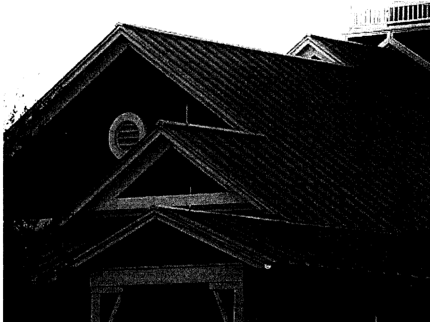
Figure 1.1b: Illustration of commonly encountered residential roofing system in Canada – Metal Roofing (Source: www.allsteel-buildings.com )
