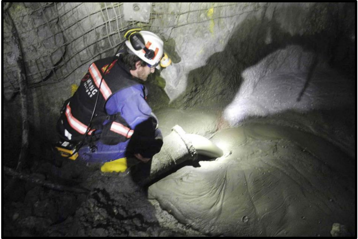
Figure 2.2: Backfilling of an underground cavity using CPB (Sika Concrete 2021)
