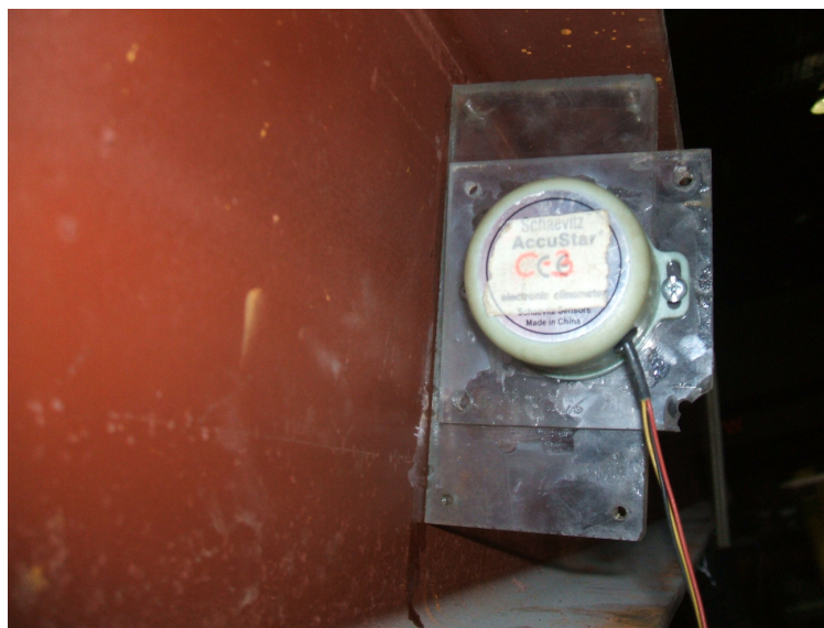
Figure 2.15-Clinometer Mounted on Gerber Beam Web at Mid-span
