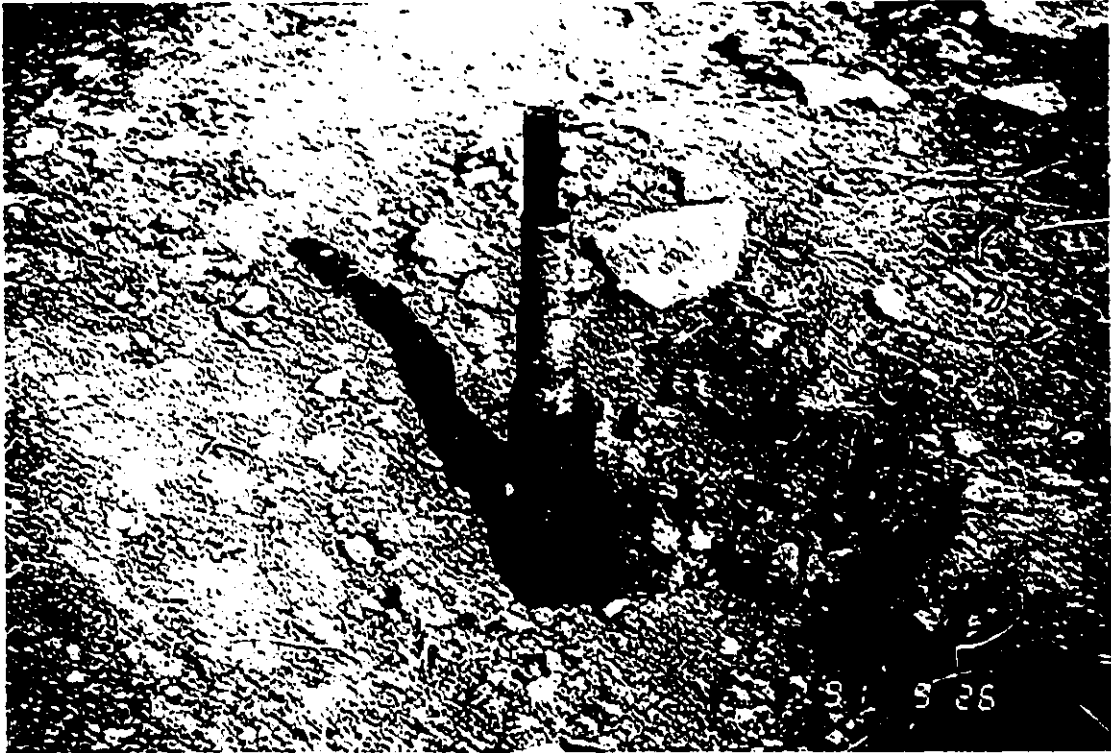
Figure 5.6 An installed heavemeter at site #1.
