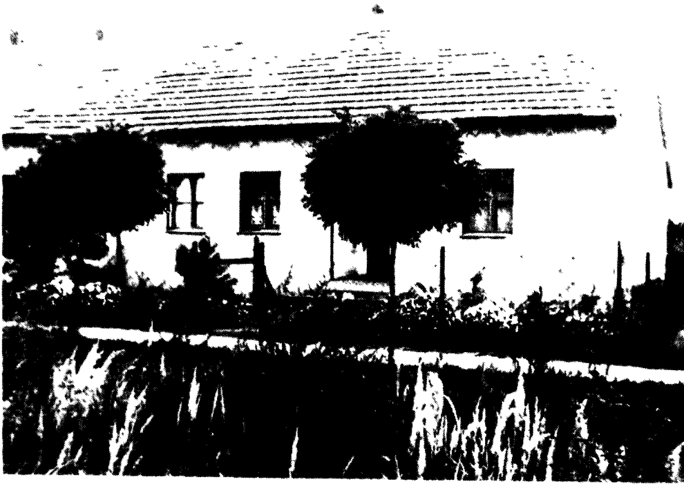
Figure 29: Nagy Berek State Farm - State Farm Worker's House
