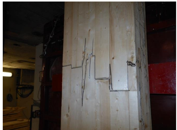
B) Tension Face Flexural Failure
