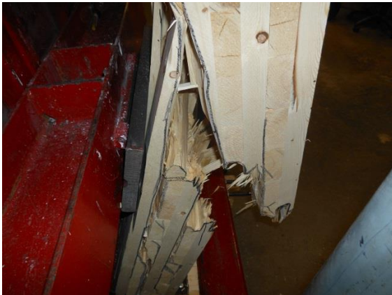
A) Left Side Flexural Failure
