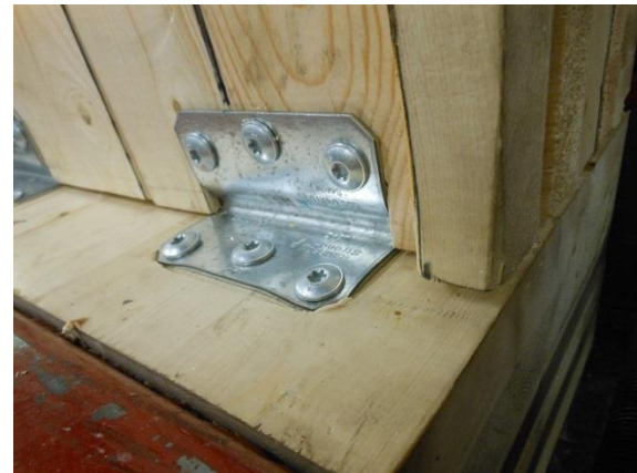
B) Embedding of Bottom Steel Angles
