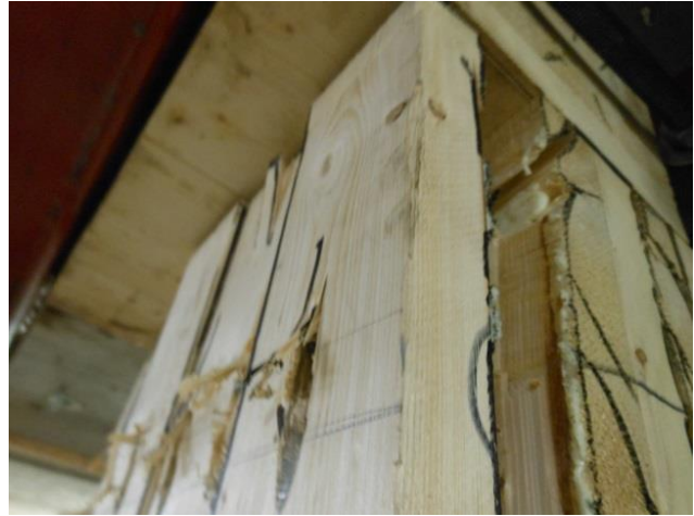
B) Close-Up of Top Failure Mode
