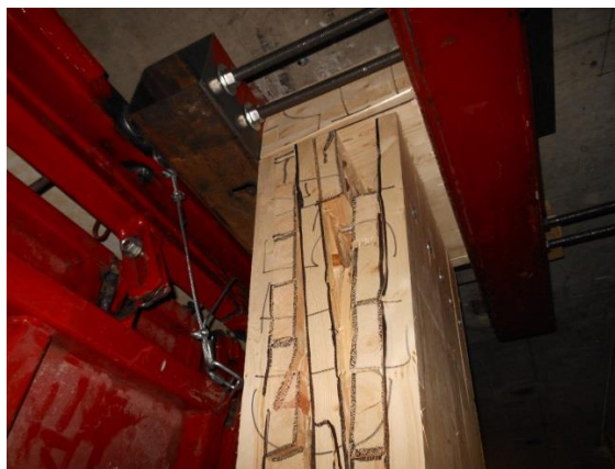
Figure 4.10: CLT 5-3 Top Connection Failure Pictures
