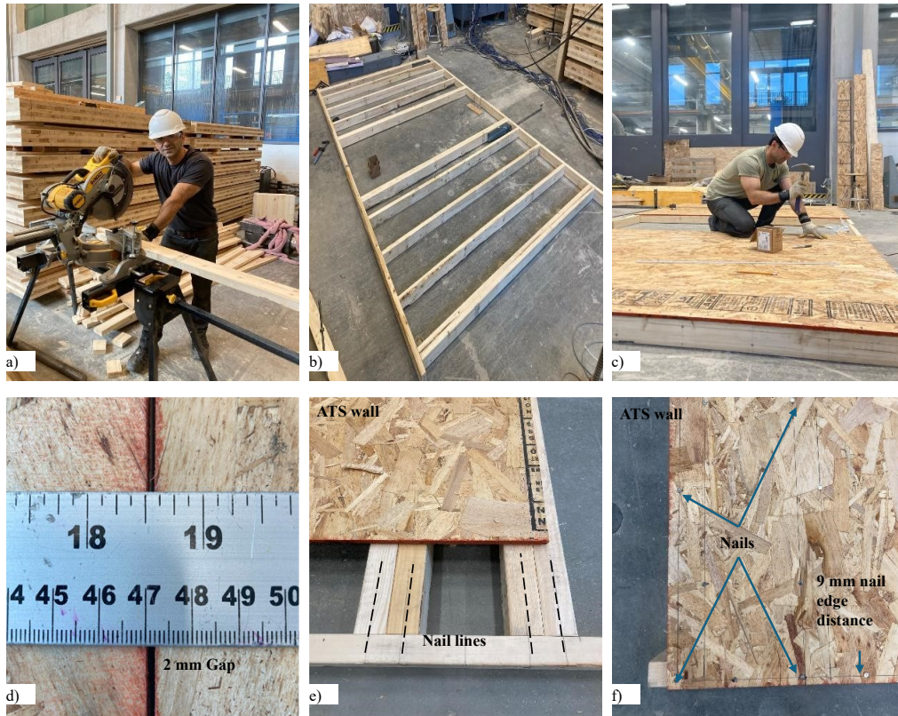
Figure 3.7: Shear wall fabrication
