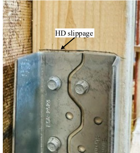
Figure 4.29: HD (HDU5) slippage in shear wall Configuration #1
