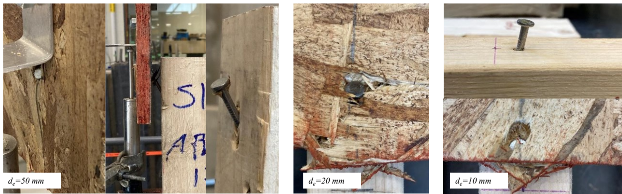
Figure 4.13: Sheathing-to-framing failure modes
