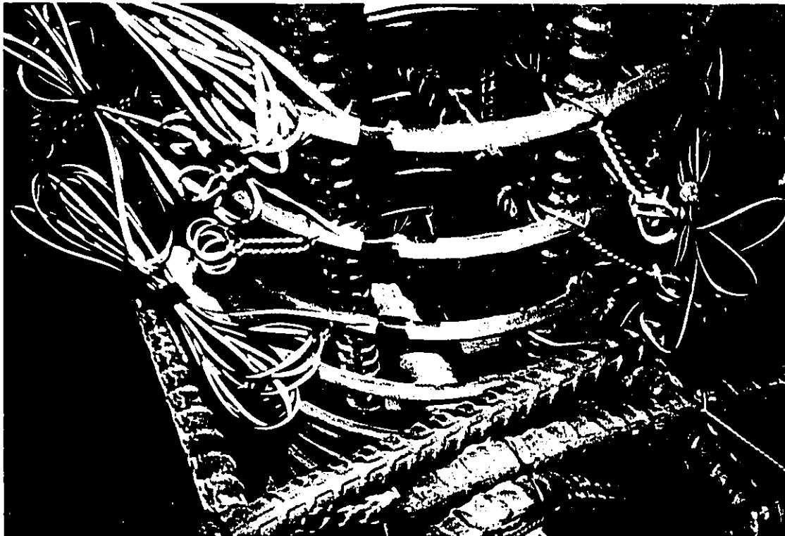
(b) Strain Gauges and Wiring on Spiral Reinforcement of a Completed Cage
