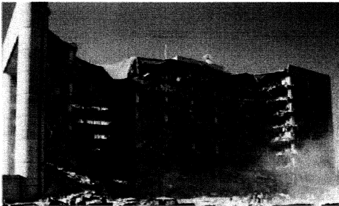
Figure 1.2: 1995 bomb attack of the Murrah Federal Building in Oklahoma City
