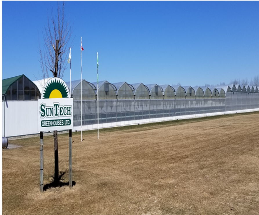
FIGURE 8.2: An outside view of deployment environment of greenhouse
