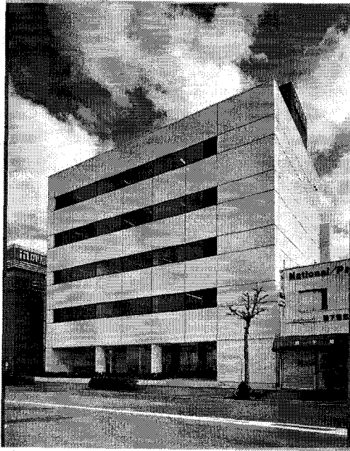
Fig. 2.5 Kajima Shizuoka Building equipped with semi-active hydraulic dampers
