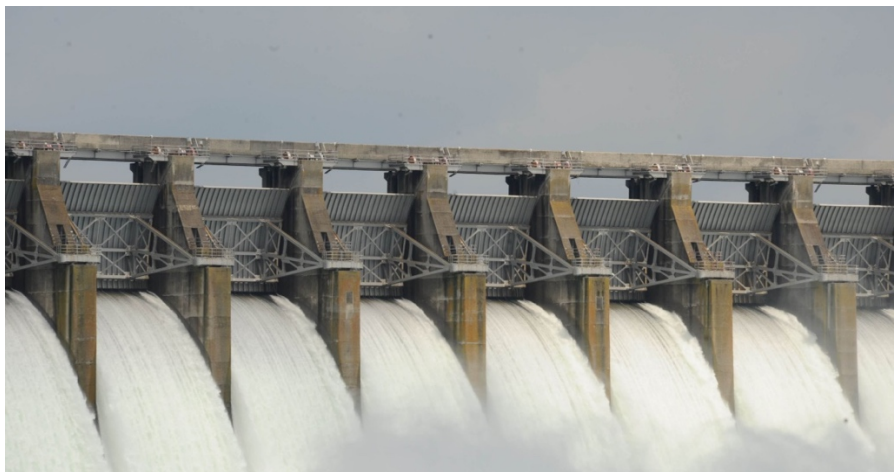
Figure 1-2 Gated spillway (The Greenville News, 2016)
