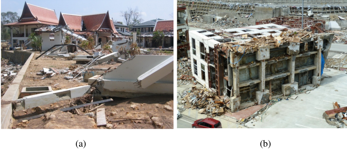
Figure 1.4. Destruction of inland structures due to tsunami-induced hydrodynamic forces: (a) 2004 Indian Ocean Tsunami, Phuket city, Thailand [CAEE, 2005]; (b) 2011 Tohoku Tsunami, Onagawa city, Miyagi prefecture, Japan [Courtesy of Dr. Ioan Nistor].
