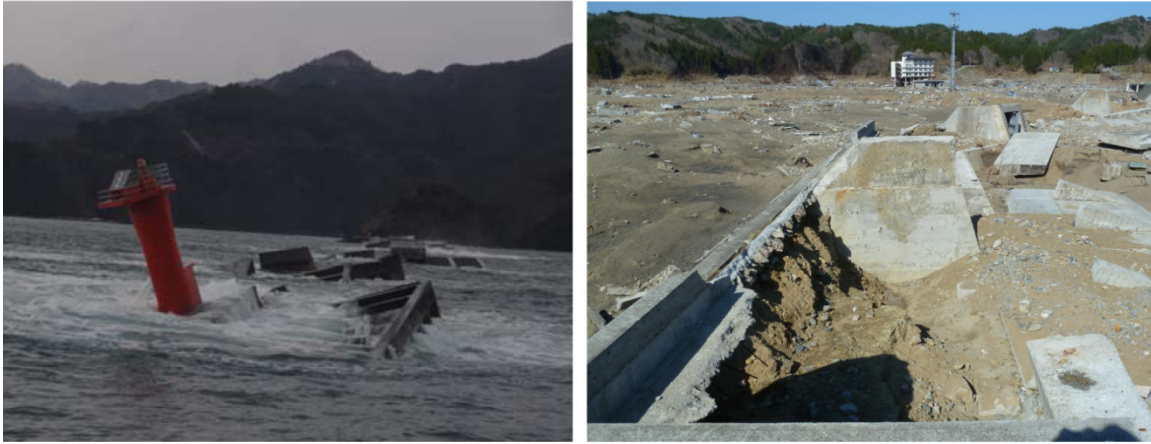
Figure 1.2. Destruction of coastal structures by the 2011 Tohoku Tsunami: (a) Overturned caissons of the breakwater at Kamaishi city, Miyagi prefecture [Takahashi et al. , 2011]; (b) Concrete panels stripped from earthen sea dike at Tarou city, Miyagi prefecture [EERI, 2011].
