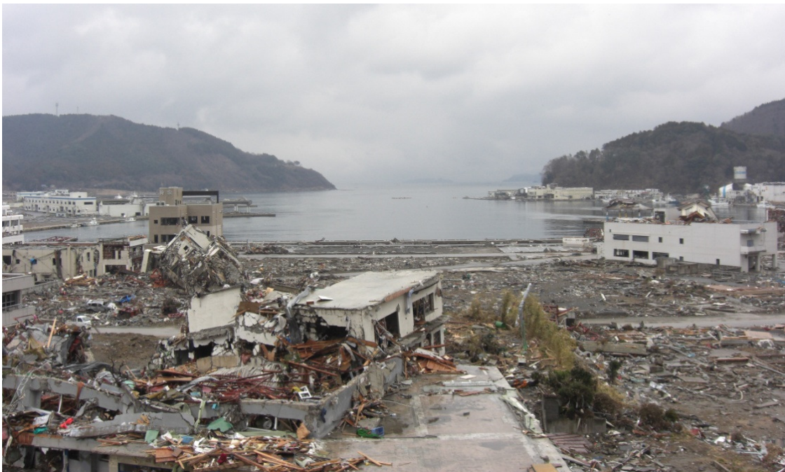
Figure 1.3. Widespread destruction of inland structures by the 2011 Tohoku Tsunami in Onagawa city, Miyagi prefecture [Courtesy of Mikami Takahito].
