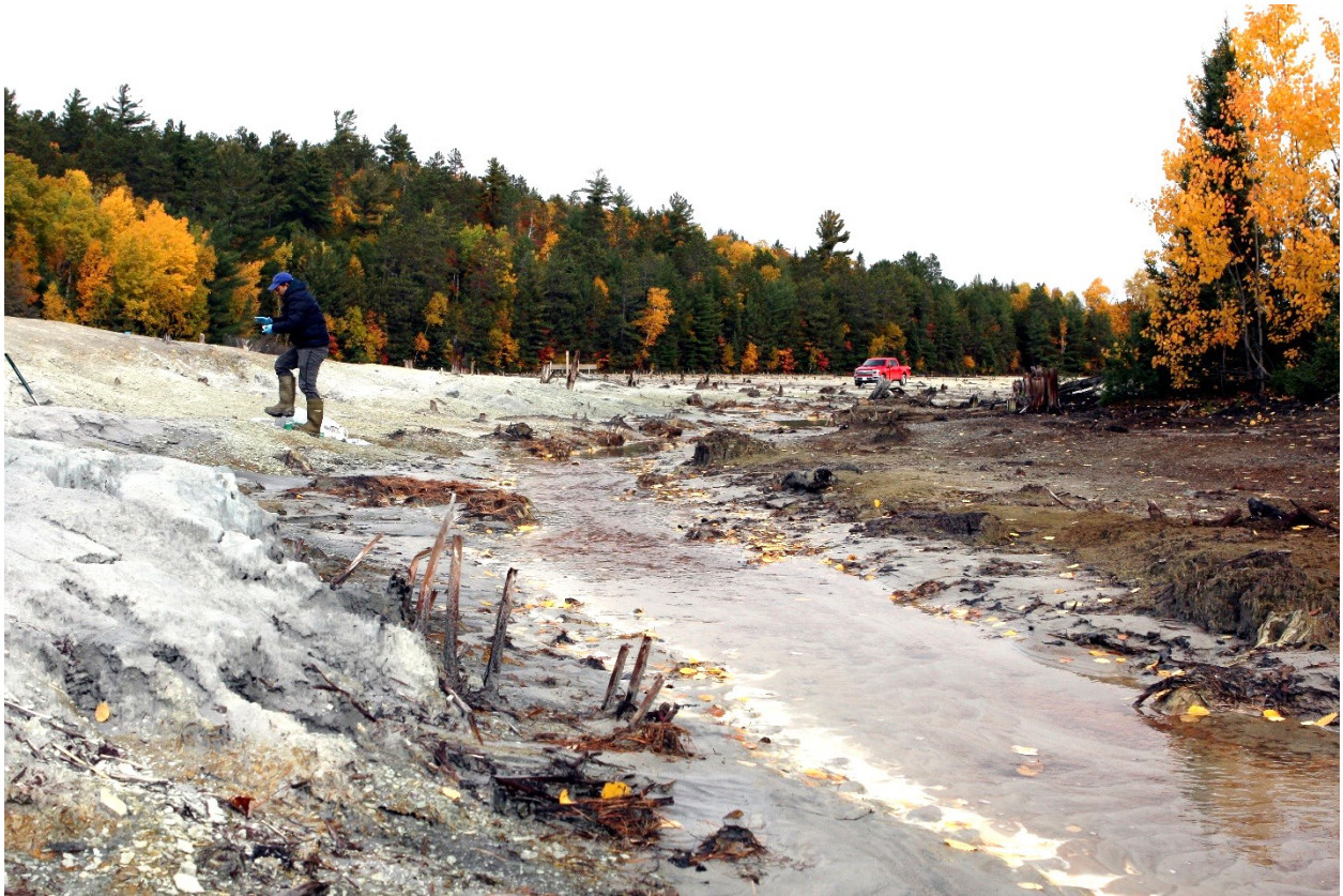
Fig. 2S.1. Tailings area TA-01(view looking north). The tailings and the cemented crusts have been eroded by the creek that flows through the tailings impoundment toward the lake.
