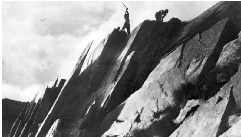
A still from Salt for Svanetia depicting the Soviet arrival and the construction of the first road in 1930s.
