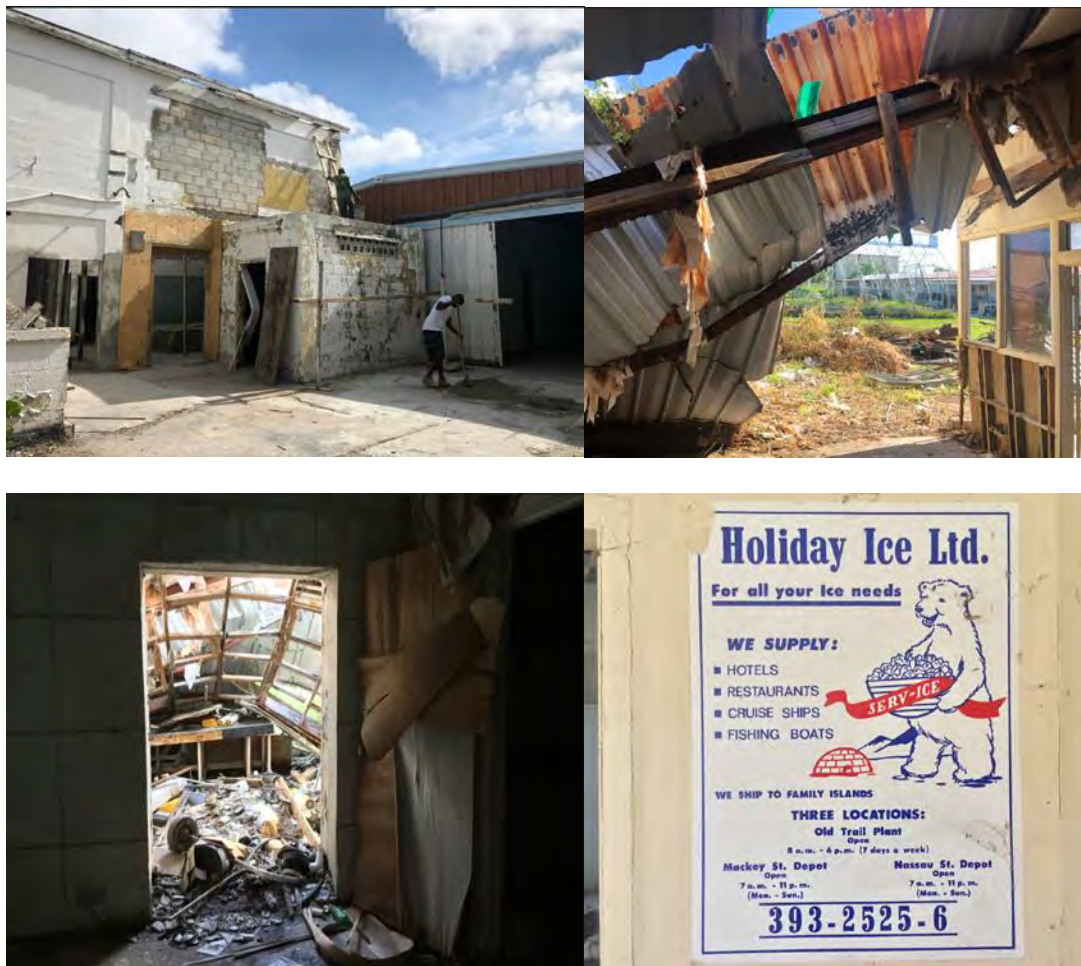
Figure 18 Renovation documentation at I.C.E.
