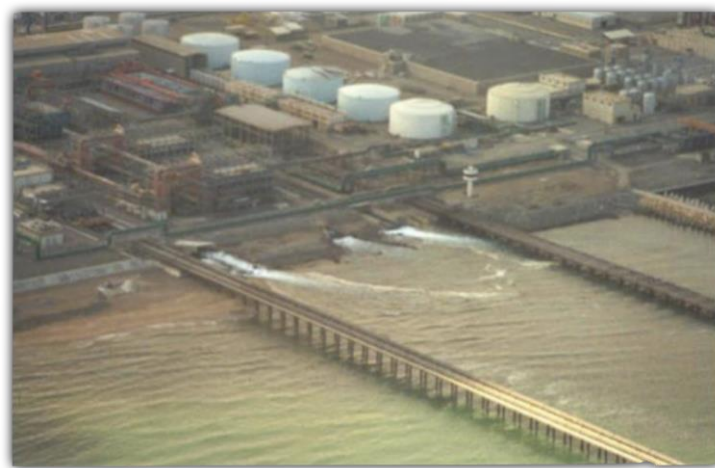
(e) Industrial wastewater
