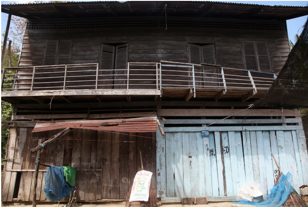
Figure 16. A boarded-up and abandoned house in Koh Kaptic village. Source: author
