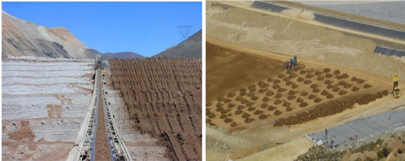
Figure 2.15. Transport of dry-stack tailings using a conveyor (left) and a truck (right) (Engels, 2002; Anglo, 2004)
