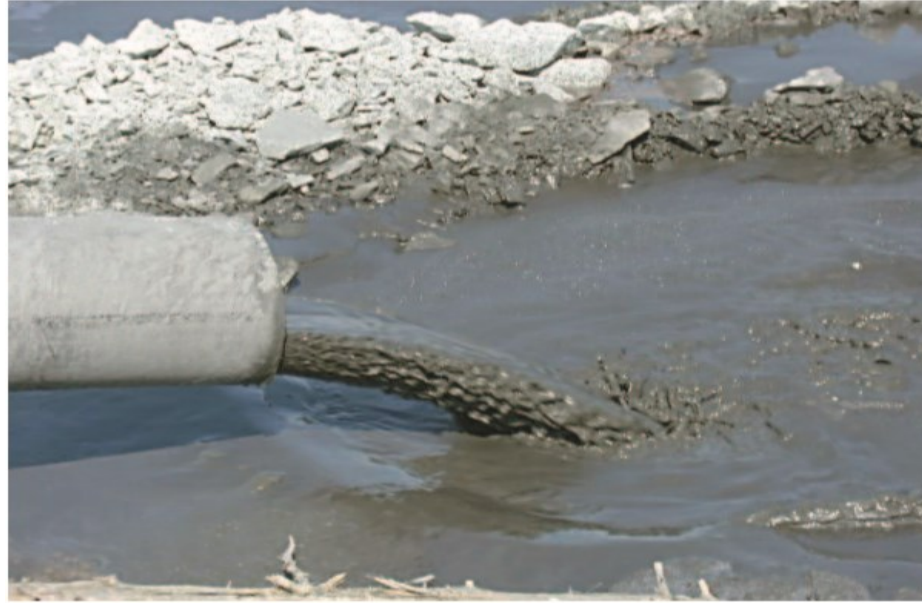
Figure 2.2. Discharging slurry tailings in a tailings impoundment (Bussière, 2007)
