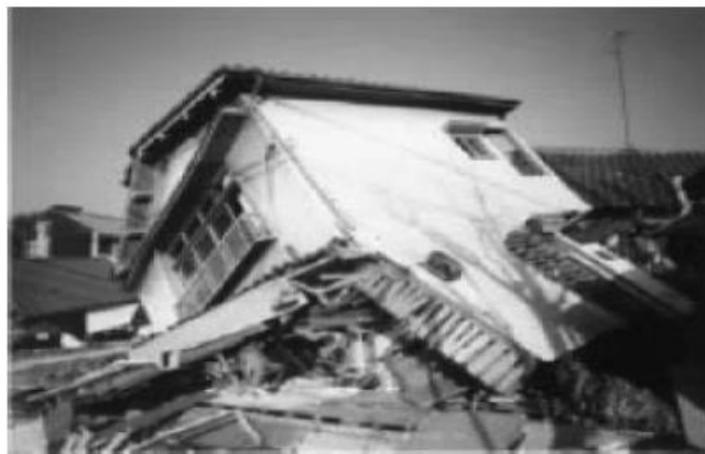
Figure 1.3: Collapse of Typical Building, 1995 Kobe Earthquake (Lam et. al 2002)
