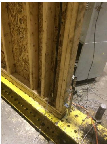
a) Tie-Rod Installation
