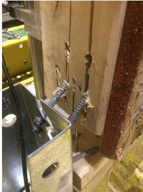
Figure 5.19: Screws Group Tear-Out Failure
