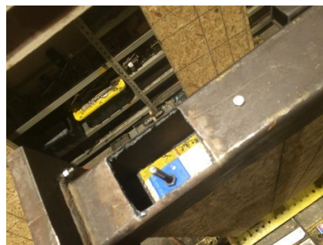
b) Bearing Plate Installation
