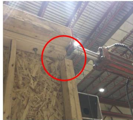
b) Nails Withdrawal at Top Plate
