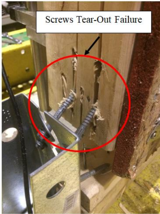
b) Hold-Down Connection Failure
