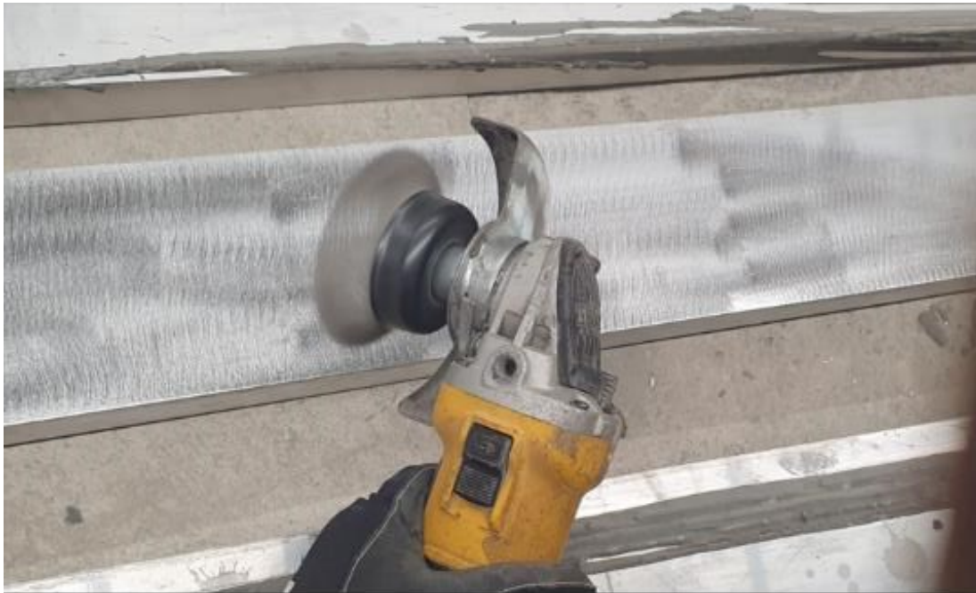
Figure 3.13: Sanding mullion surface by a metal brush specific for aluminum surfaces
