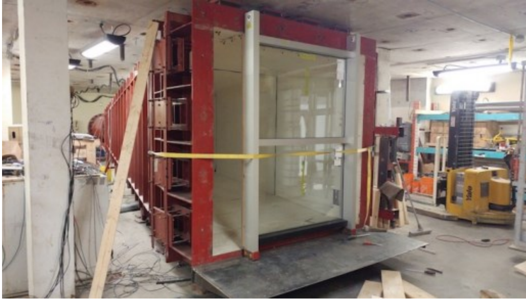
Figure 2.35: Installation of curtain wall specimen (Saatcioglu et al., 2017a)
