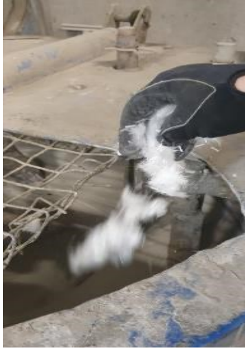
Figure 3.26: PVA fibers gradually added to ECC mix
