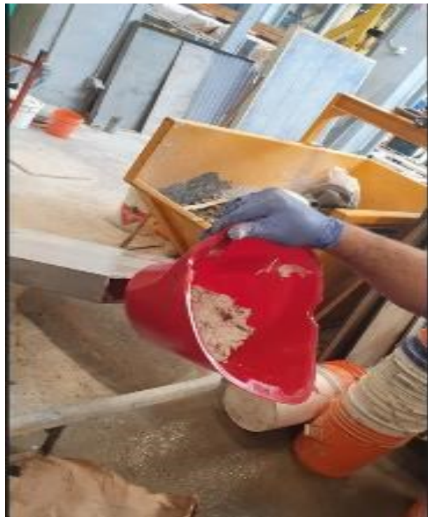
Figure 3.27: Pouring material into the mullion using a plastic funnel
