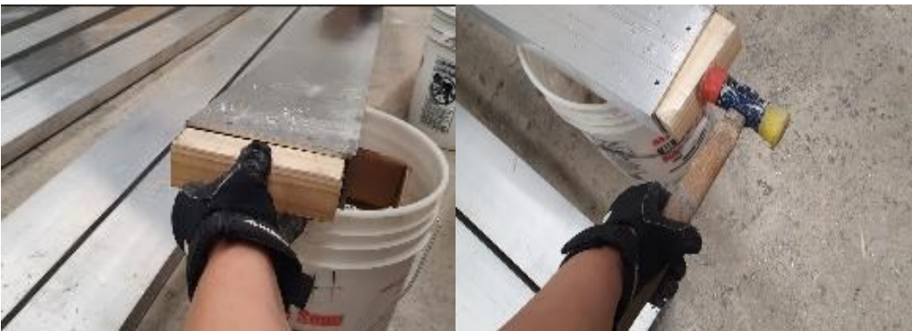
Figure 3.2: Closing mullion end by a wooden block
