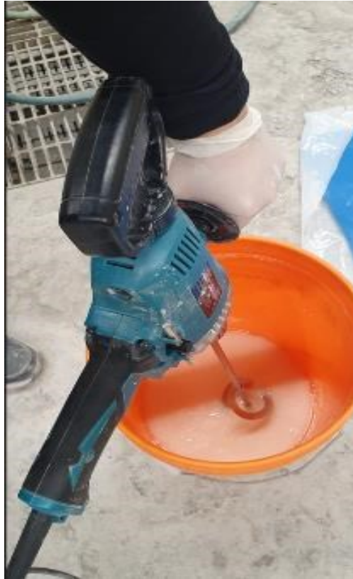
Figure 3.18: Epoxy mixing process using a hand mixer
