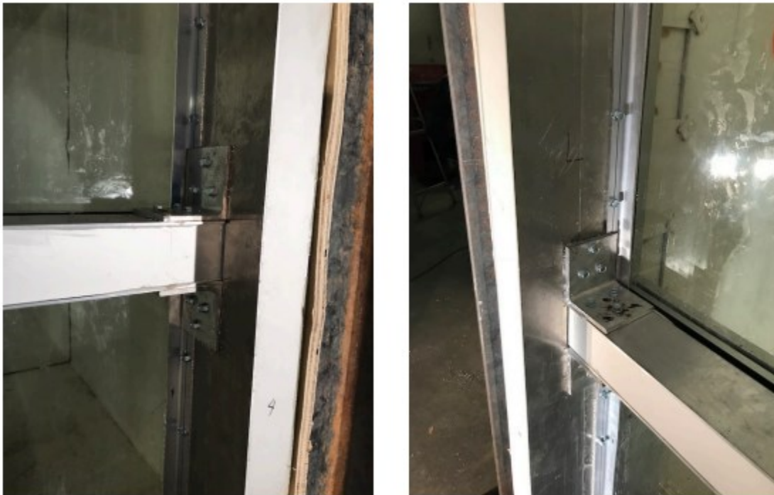
Figure 2.46: Mechanical glazing and mullion connection strengthening (Saatcioglu, 2020)
