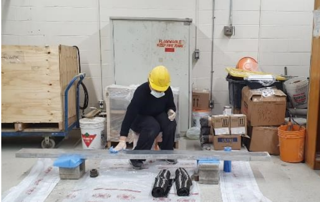
Figure 3.14: Mullion surface cleaning prior to CFRP application
