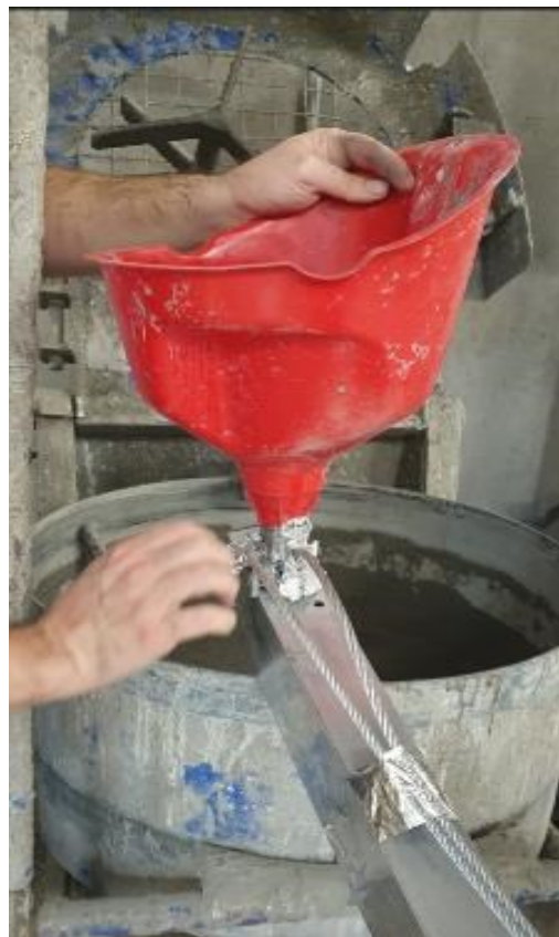
Figure 3.7: Material pouring into the mullion by using a plastic funnel
