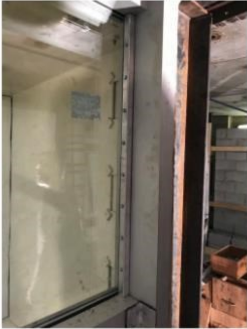
(a) Mechanical glazing
