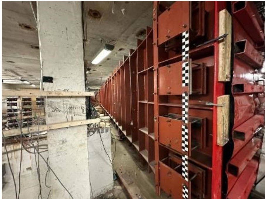
Figure 3.49: Square vents close to shock-tube opening
