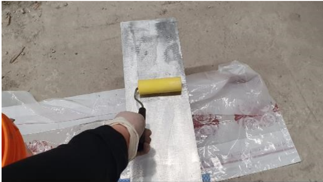
Figure 3.15: Epoxy application by a paint roller
