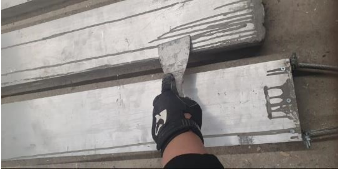
Figure 3.12: Mullion surface cleaning from the excess materials
