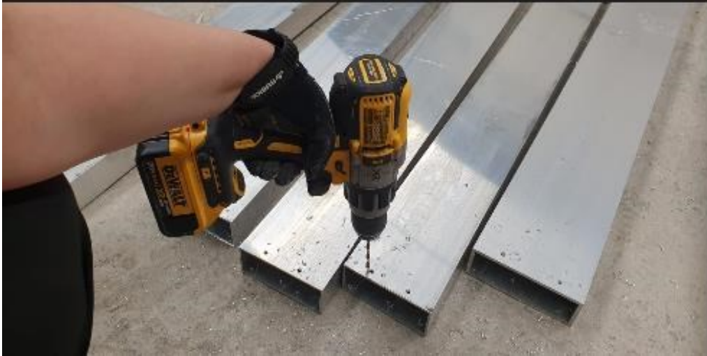
Figure 3.1: Hole drilling at mullion ends
