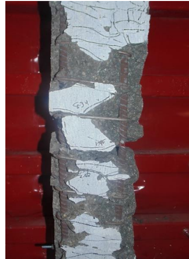
h) Tension face and bar rupture at blast 5
