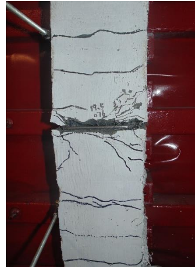
f) Tension Face After blast 3
