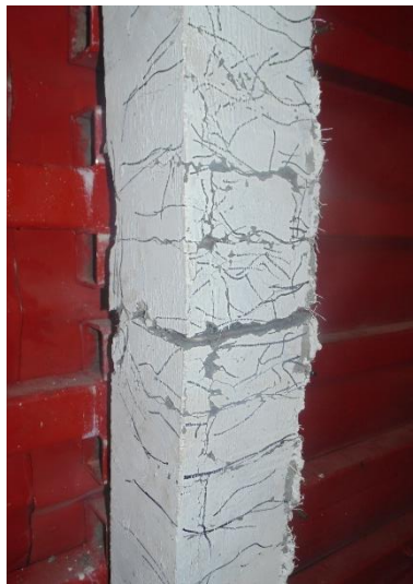
g) Mid-span at blast 5
