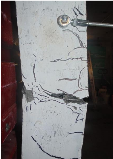
d) Mid-span After blast 3
