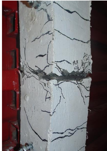
e) Mid-span After blast 3
