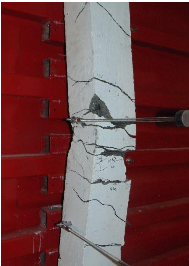
d) Mid-span at blast 3
