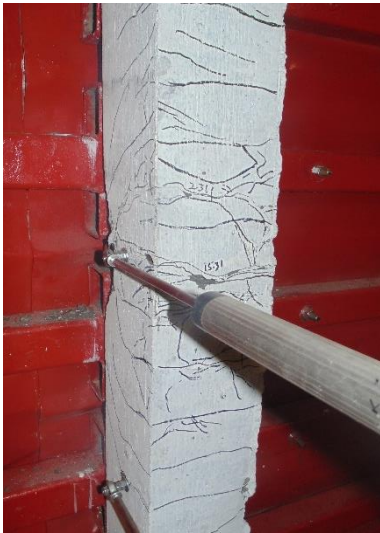
e) Tension face at blast 3
