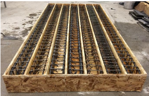
f) Prior to casting
