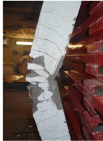
g) Mid-span at blast 4
