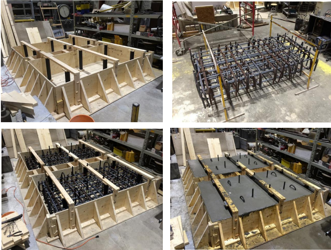
Figure 103.25 Construction process of footings
