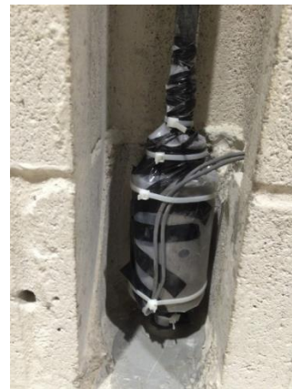
Figure 113.35 (a) Post-tensioning strand and anchor (covered by plastic) prior to concrete placement
