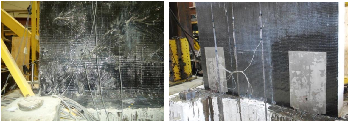
Figure 2.26 Installed FRP and ductile steel sheet anchors on PRM and URM walls, respectively
