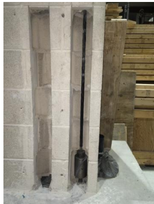
Figure 113.35 (a) Post-tensioning strand and anchor (covered by plastic) prior to concrete placement
