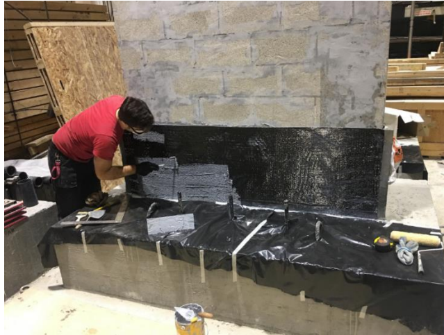
Figure 119.40 First layer of carbon FRP (SikaWrap-230 C) being attached on masonry wall
