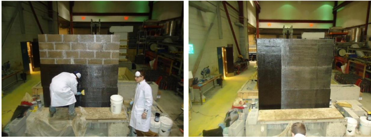
Figure 2.25 Application of FRP sheets on masonry wall
