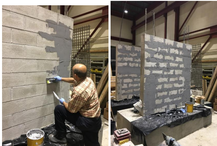
Figure 117.38 Sikadur 30 epoxy mortar was used to fill irregularities and bed joints
