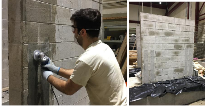
Figure 116.37 Masonry wall surface made level and clean by grinding and washing
