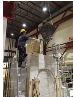
Figure 110.32 Left: Casting of concrete inside the masonry wall cells, Right: Masonry wall ducts after casting of concrete
