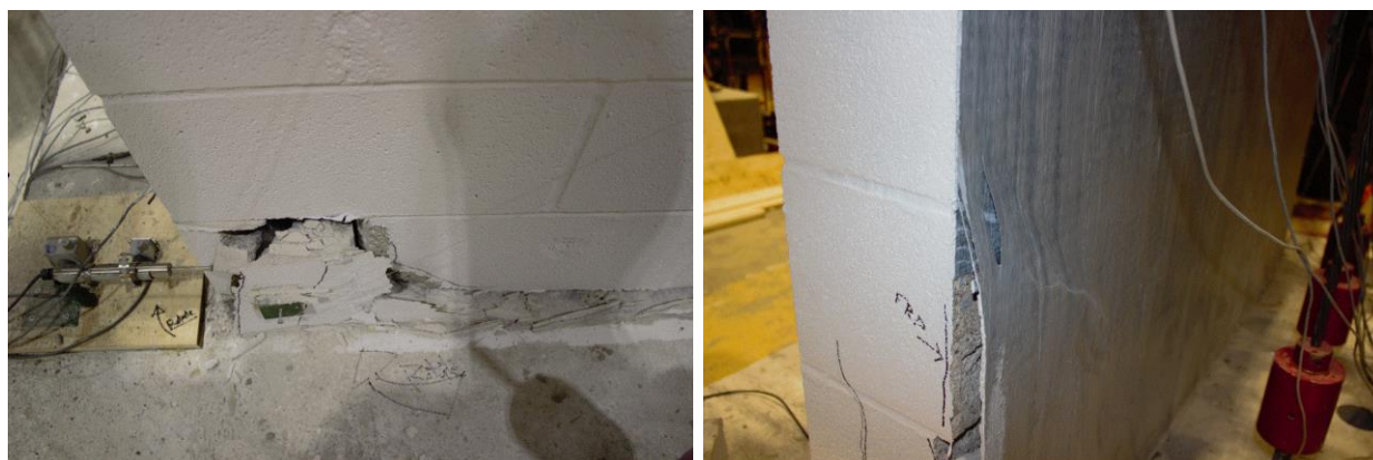
(a) Rotation of east end towards north
