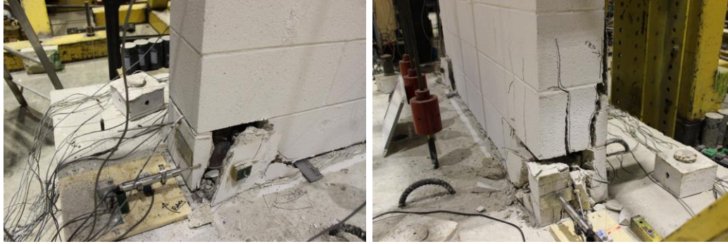
Figure 163.28 Damage progress of wall 2 at toe regions, 1.25% drift
