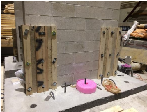
Figure 109.31 Installation of formworks on top of the open ducts by bolts
