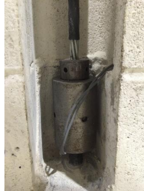
Figure 112.34 Post-tensioning cable secured at its place between to prestressing anchors
