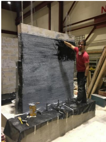
Figure 120.41 Installation of horizontal and vertical layers of FRP sheets
