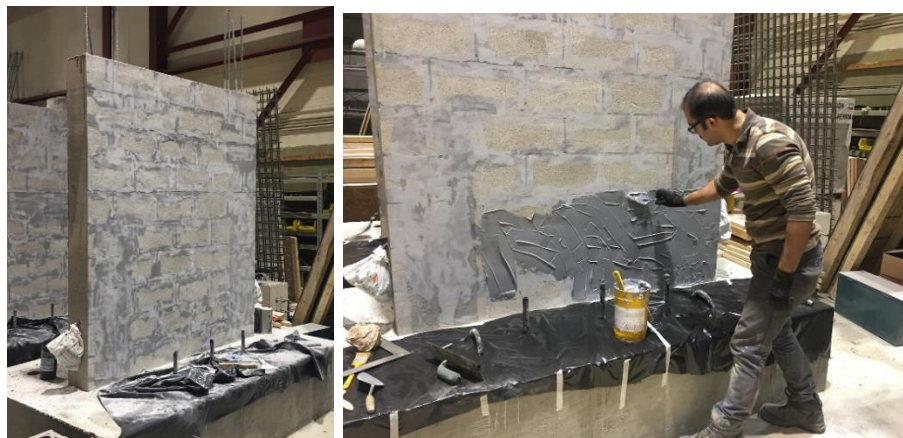
Figure 118.39 (a) dried epoxy mortar was grinded to create smooth surface fore FRP attachment, (b) Sikadur 330 epoxy glue applied on top of the wall for FRP attachment
