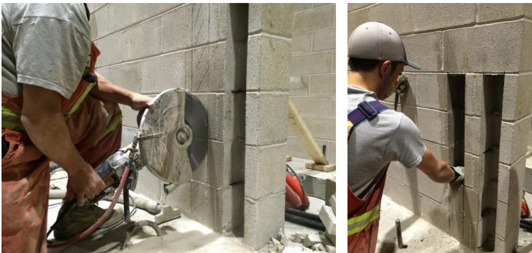
Figure 105.27 Cutting of masonry walls to create open ducts
