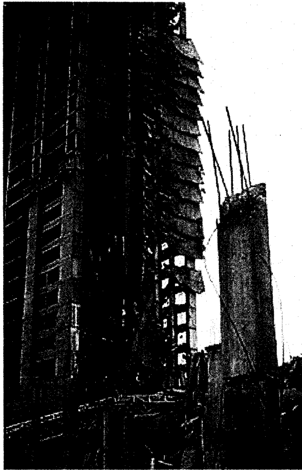
Figure 1.3: Construction failure, Bailey's Crossroads, Fairfax, Virginia, March 1973. Photo courtesy of the National Institute of Standards and Technology
