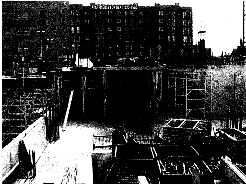
Figure 1.2: Flat slab building under construction with 1 level of scaffold shoring combined with flying forms
