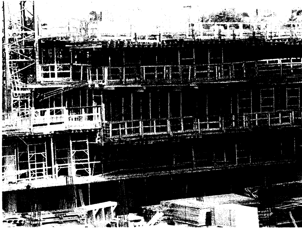
Figure 1.1: Flat slab building under construction with 3 levels of scaffold shoring and 1 level of reshores (bottom level)
