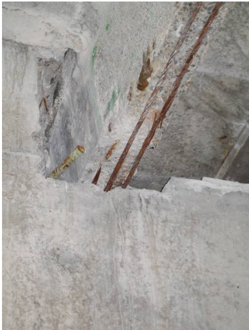
Figure 4-11: Corrosion-induced damage in the soffit of girders in a parking garage structure in Ottawa
