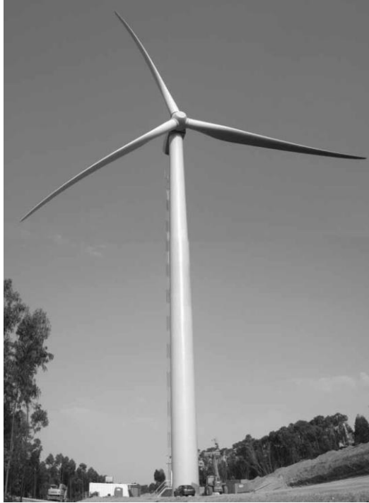
Figure 2.1 Steel tubular tower (Veljkovic et al., 2011)
