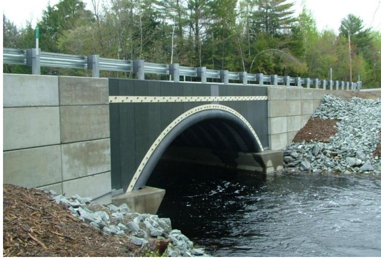
Figure 2.7 Buried CFFT arch bridge in Bradley, Maine, USA (constructed in 2010) (Dagher et al., 2012)
