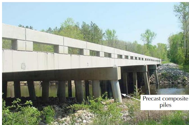
Figure 2.6 Route 40 Bridge over the Nottoway River in Virginia (Fam et al., 2003)
