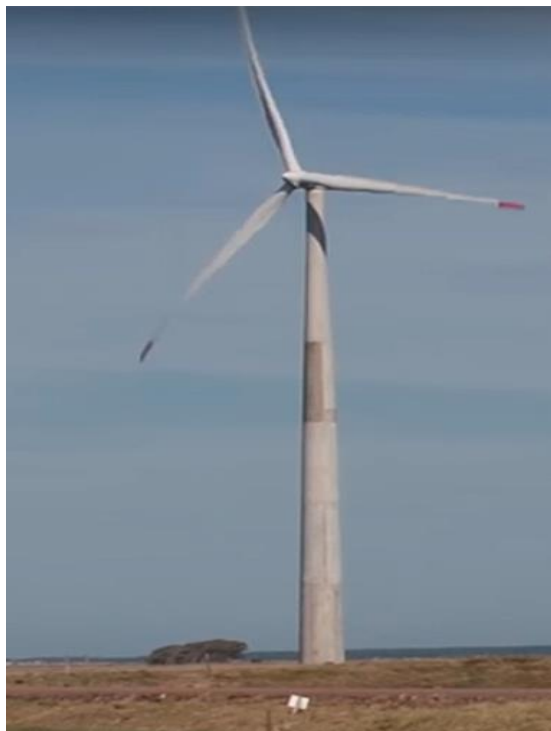
Figure 2.2 Concrete tower (ACCIONA, n.d.)
